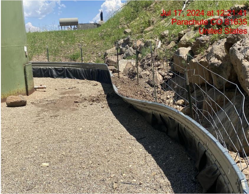
Damaged Berm from Destabilized Cut Slope – Photo #02299
