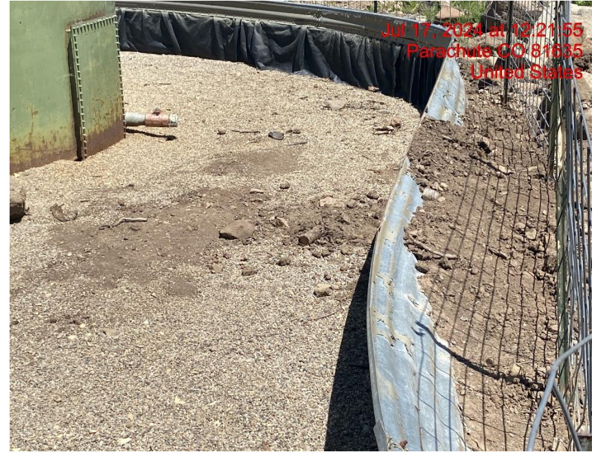
Damaged Berm from Destabilized Cut Slope – Photo #02300
