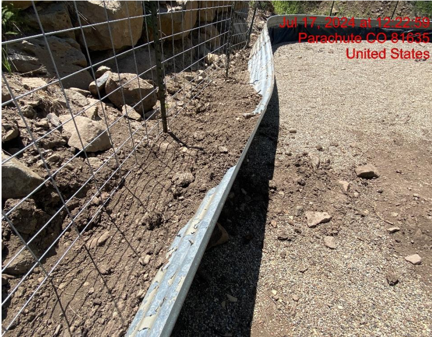
Damaged Berm from Destabilized Cut Slope – Photo #02301
