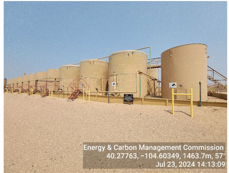
Photo 4: Tank Battery
