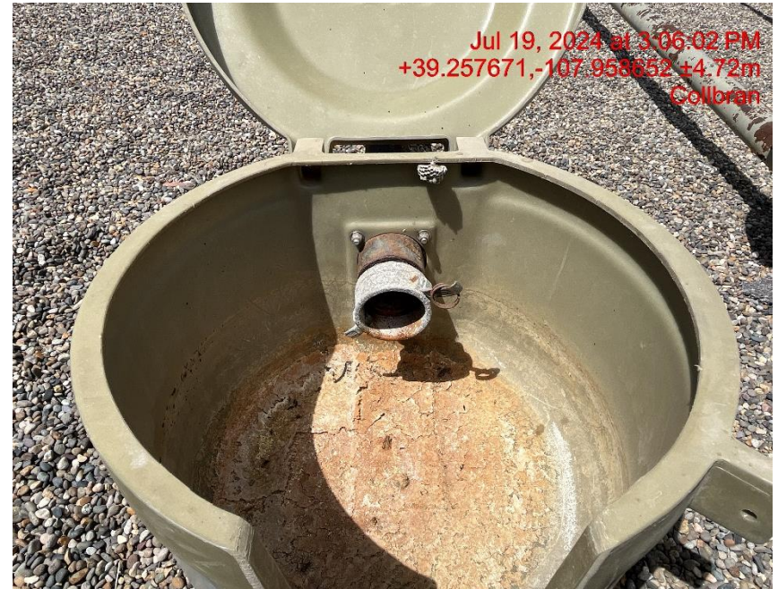
Open ended load line - Photo #03561
