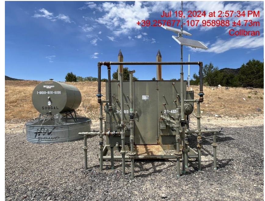
Separators/Methanol tank - Photo #03550
