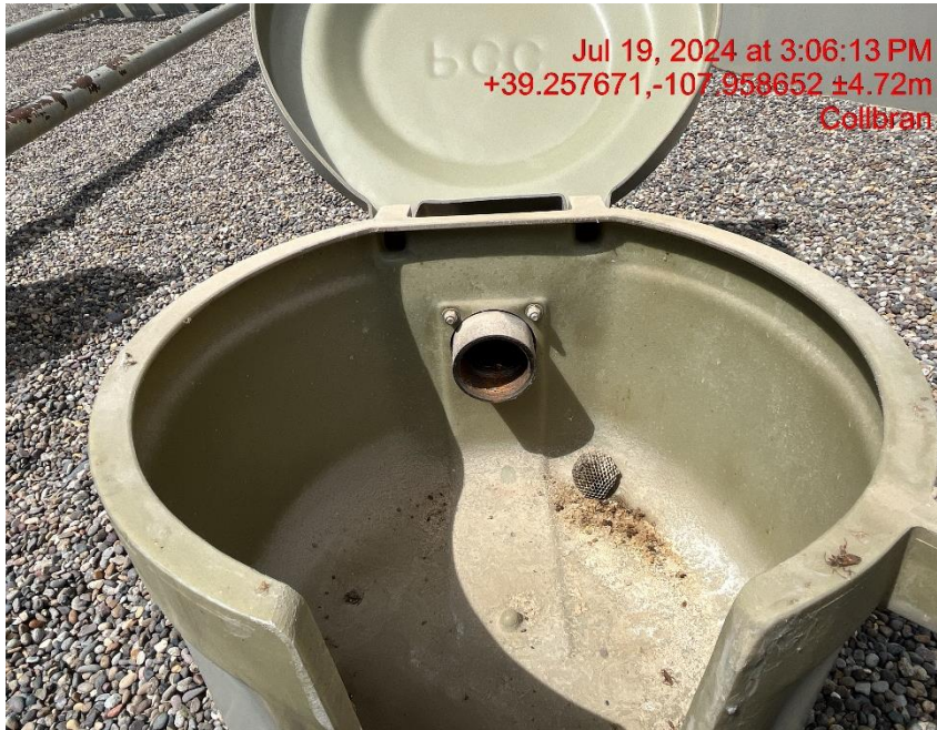
Open ended load line - Photo #03562
