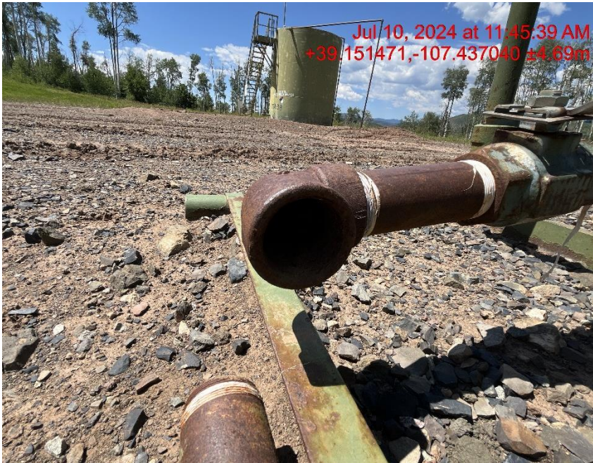
Open ended piping/wildlife hazard - Photo #03484
