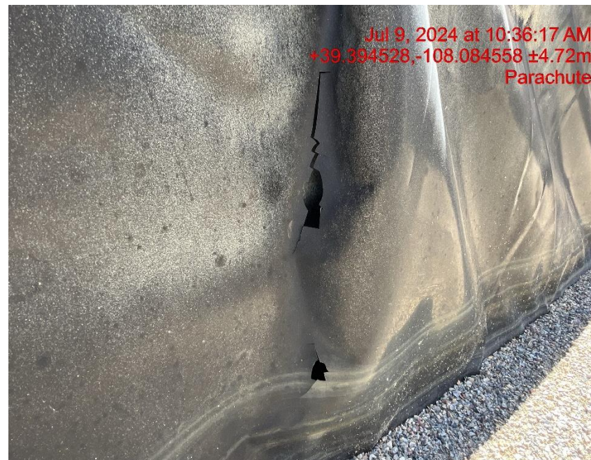
Holes in containment liner - Photo #03398
