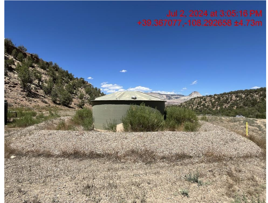
Tank Battery/Berm permeability is inadequate due to weed growth in berm - Photo #03305
