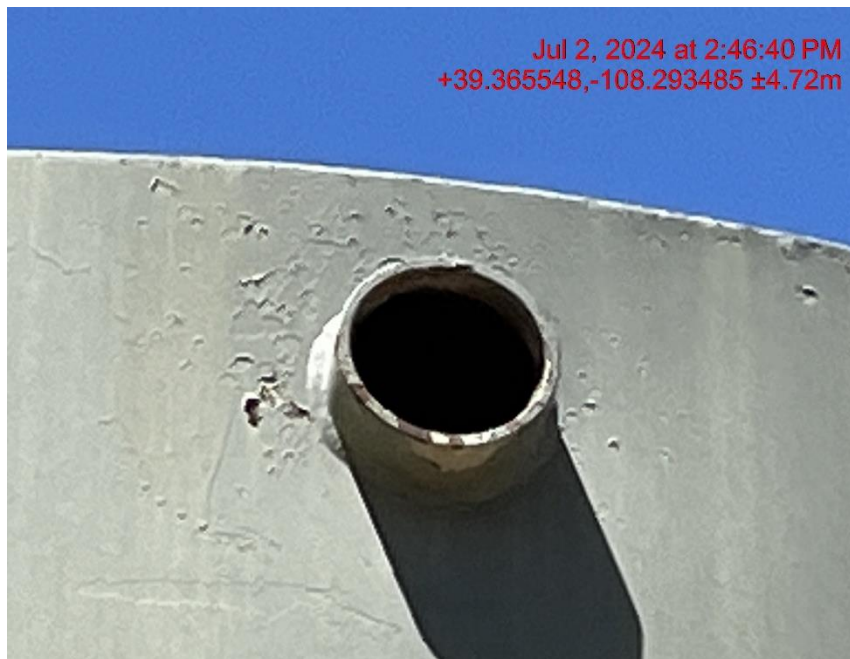
Tank port open entry to wildlife hazard - Photo #03288
