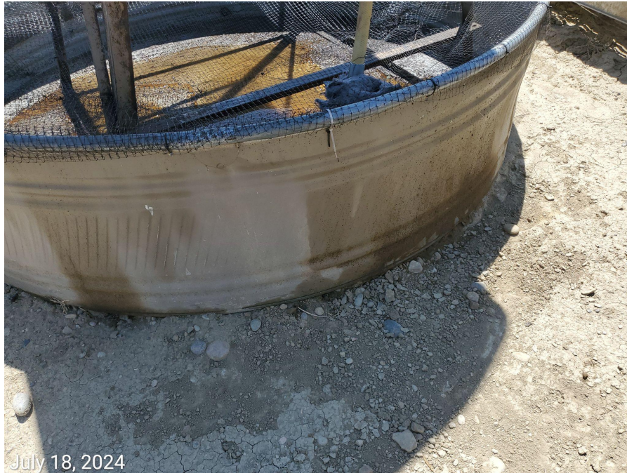
Photo 2: Stained soils at/beneath methanol tank remains evident.
