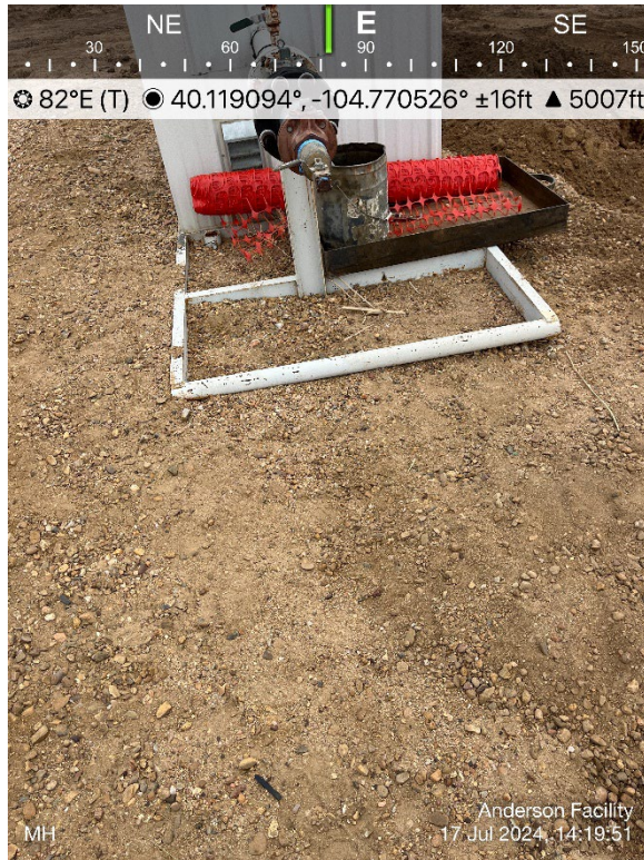
Meter House Location
