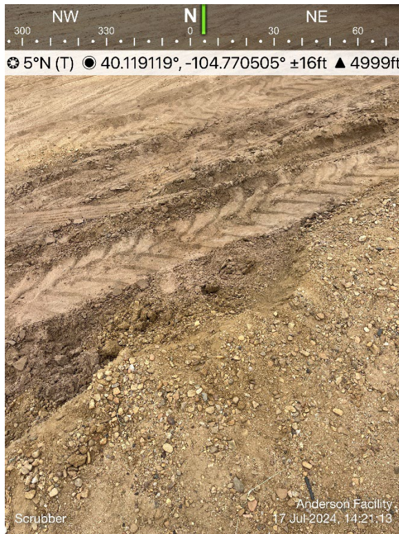
Separator Scrubber Location
