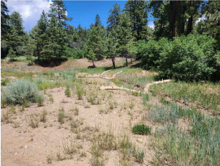
Install erosion logs in drainage
