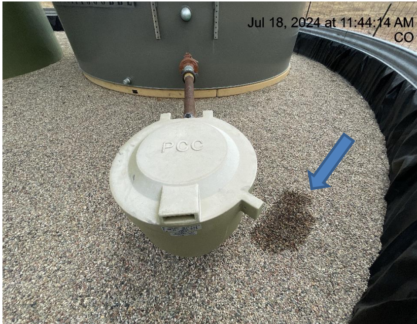
Photo # 3021 Small amount of staining in secondary containment
