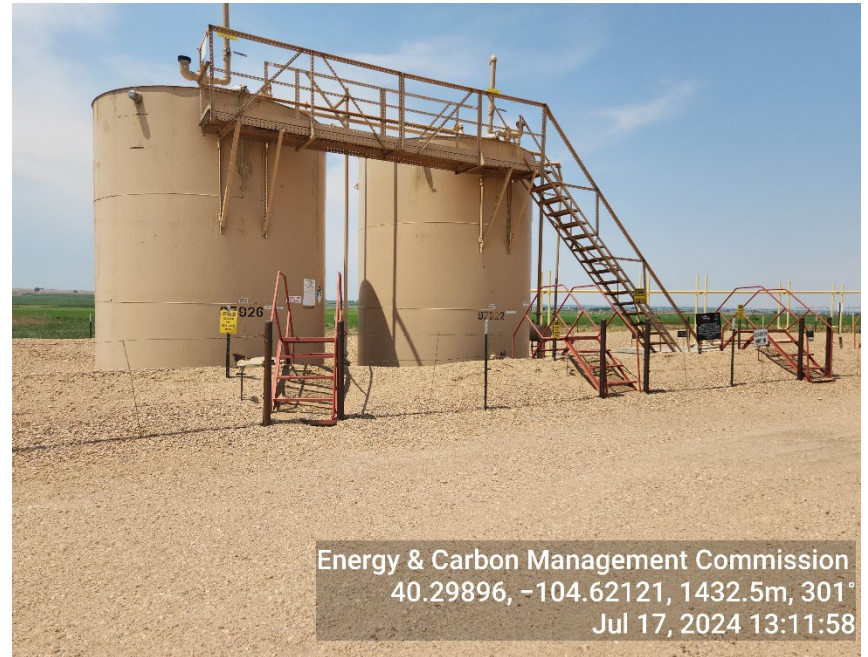
Photo 2: Tank Battery
