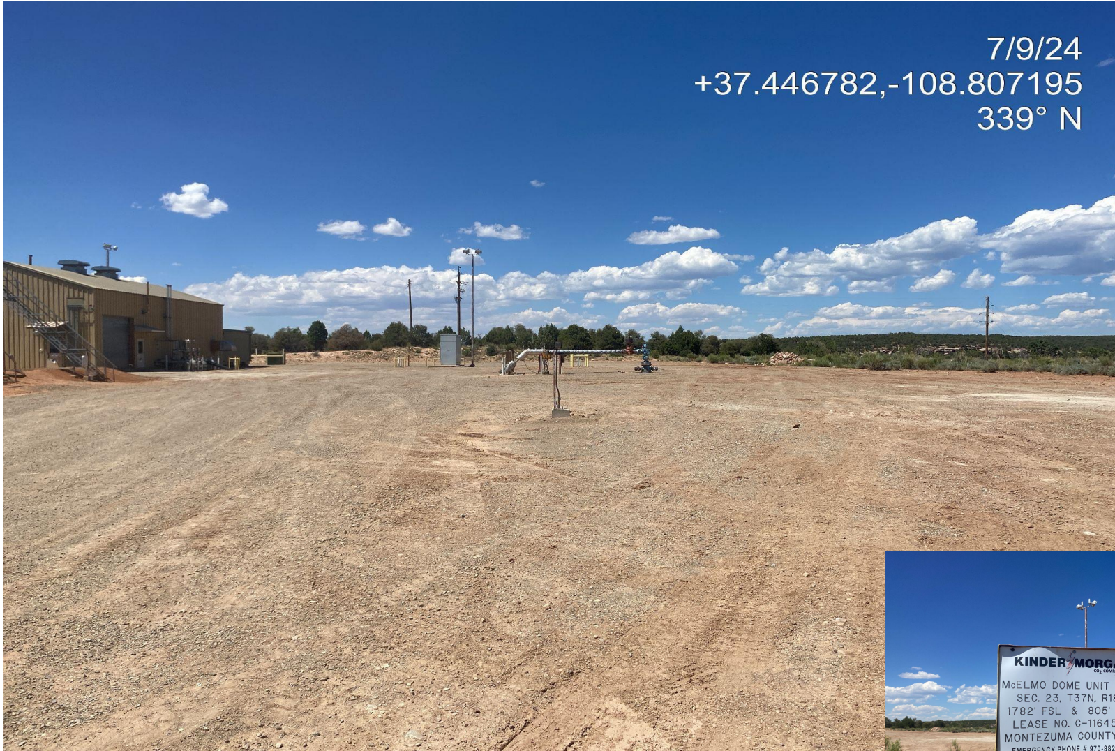
Photo 1. View of the well pad taken from the access point facing center.
