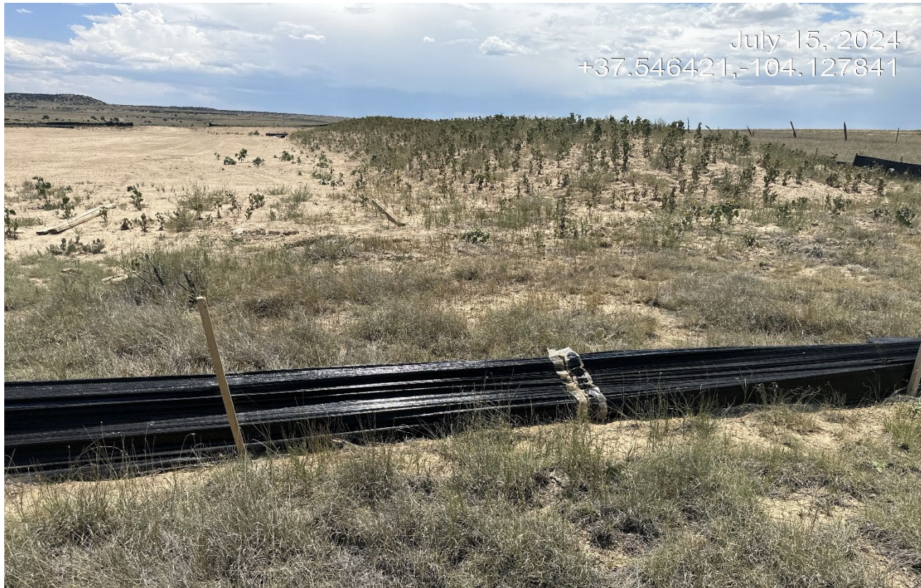
Photo 9. Southwest side of the location facing east. The silt fence is down and not maintained.
