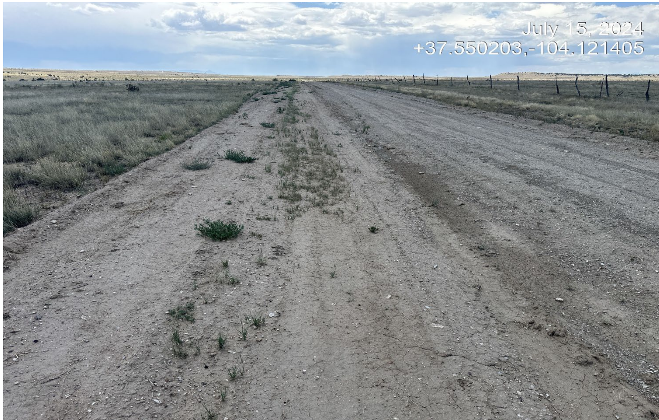
Photo 1. Facing south toward the access road. The sides of the road will need to be reclaimed. The road has been regraded and crowned since previous inspection.
