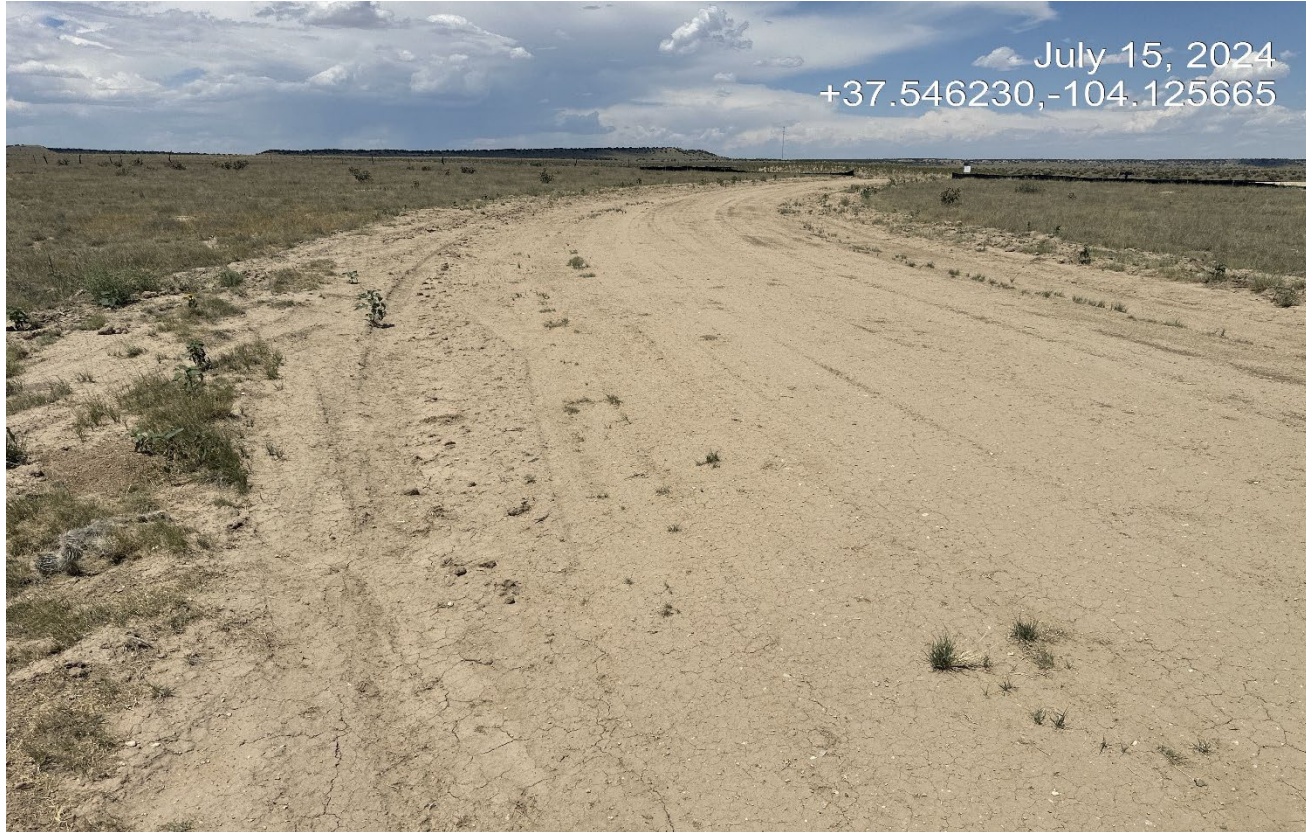
Photo 3. Facing northwest toward the access road. The side of the road needs to be seeded and stabilized. Previous corrective action was not completed.
