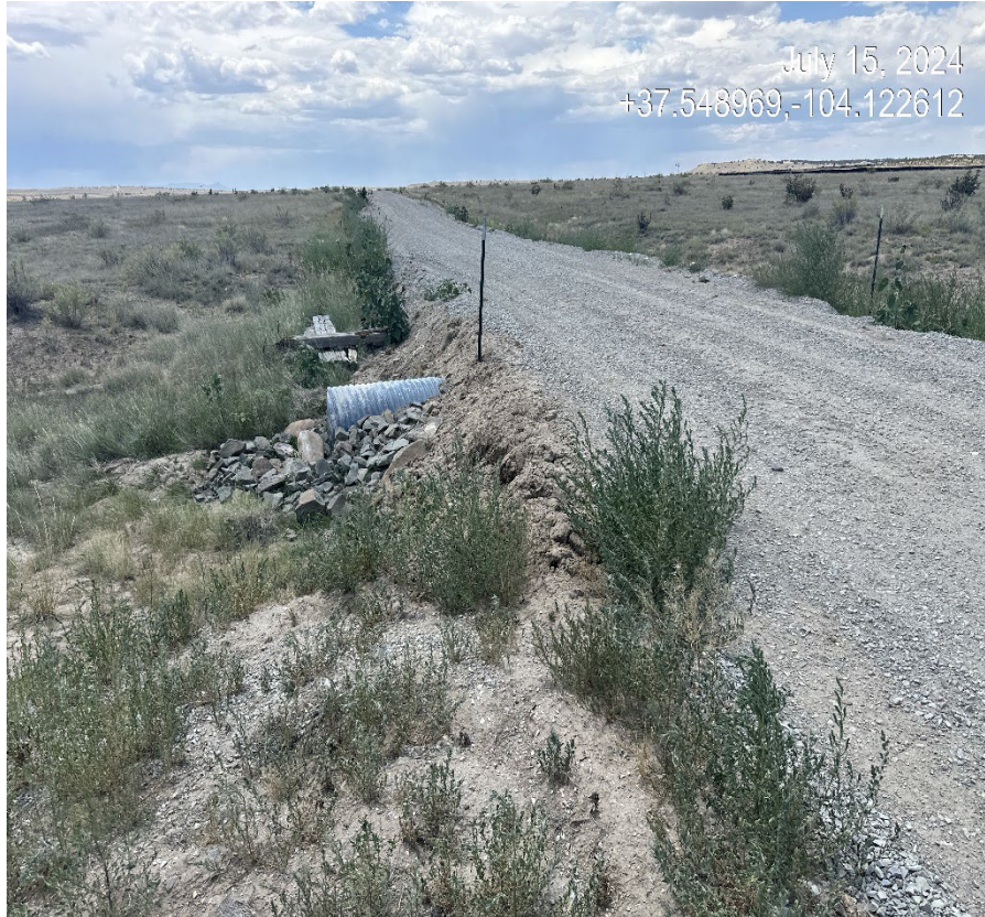
Photo 2. The culvert outlet has been repaired and outlet protection was installed, The loose soil along the embankment need to be stabilized..
