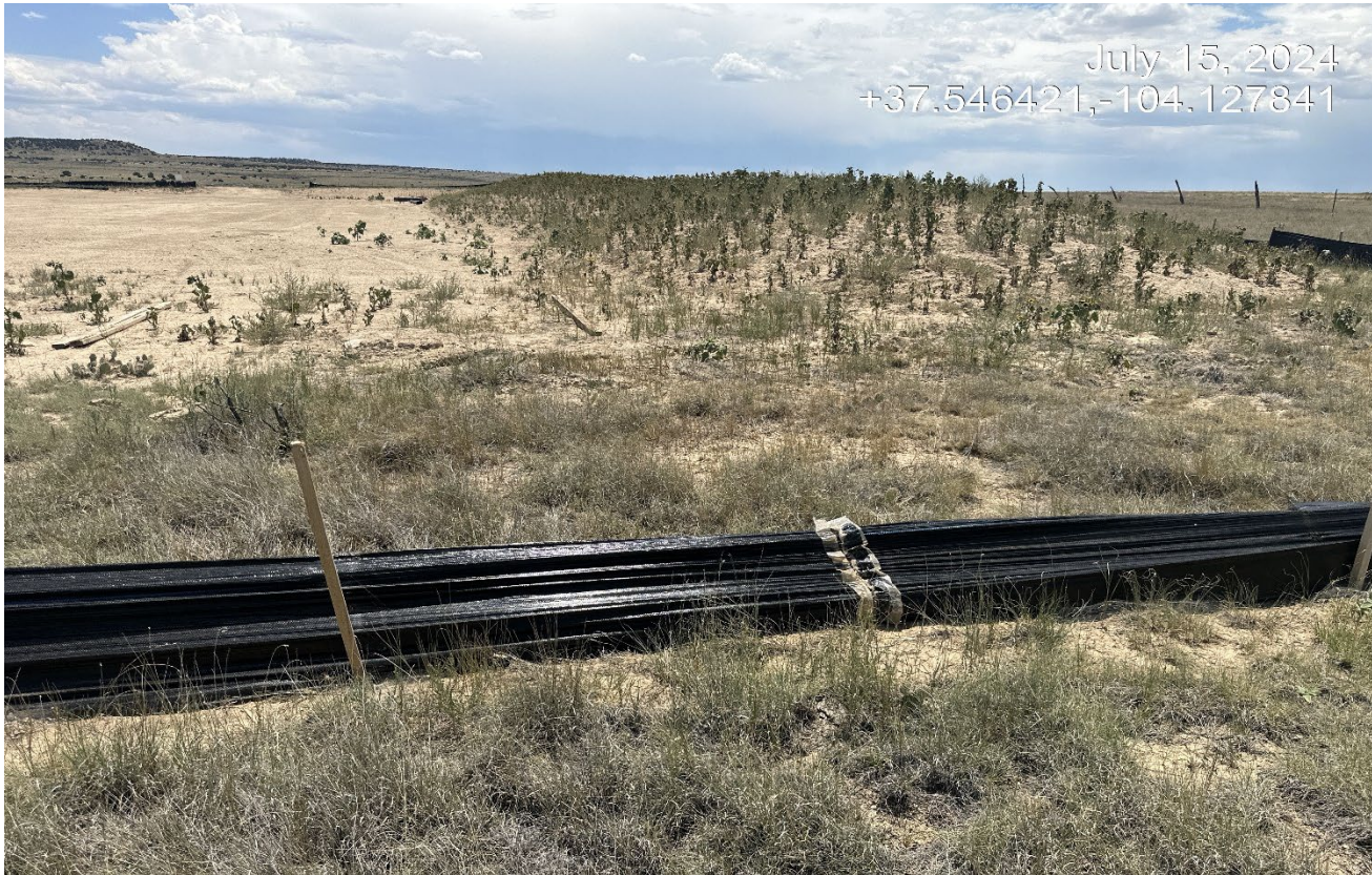
Photo 7. Facing toward the drilled well which has a steel grate to prevent wildlife entry.
