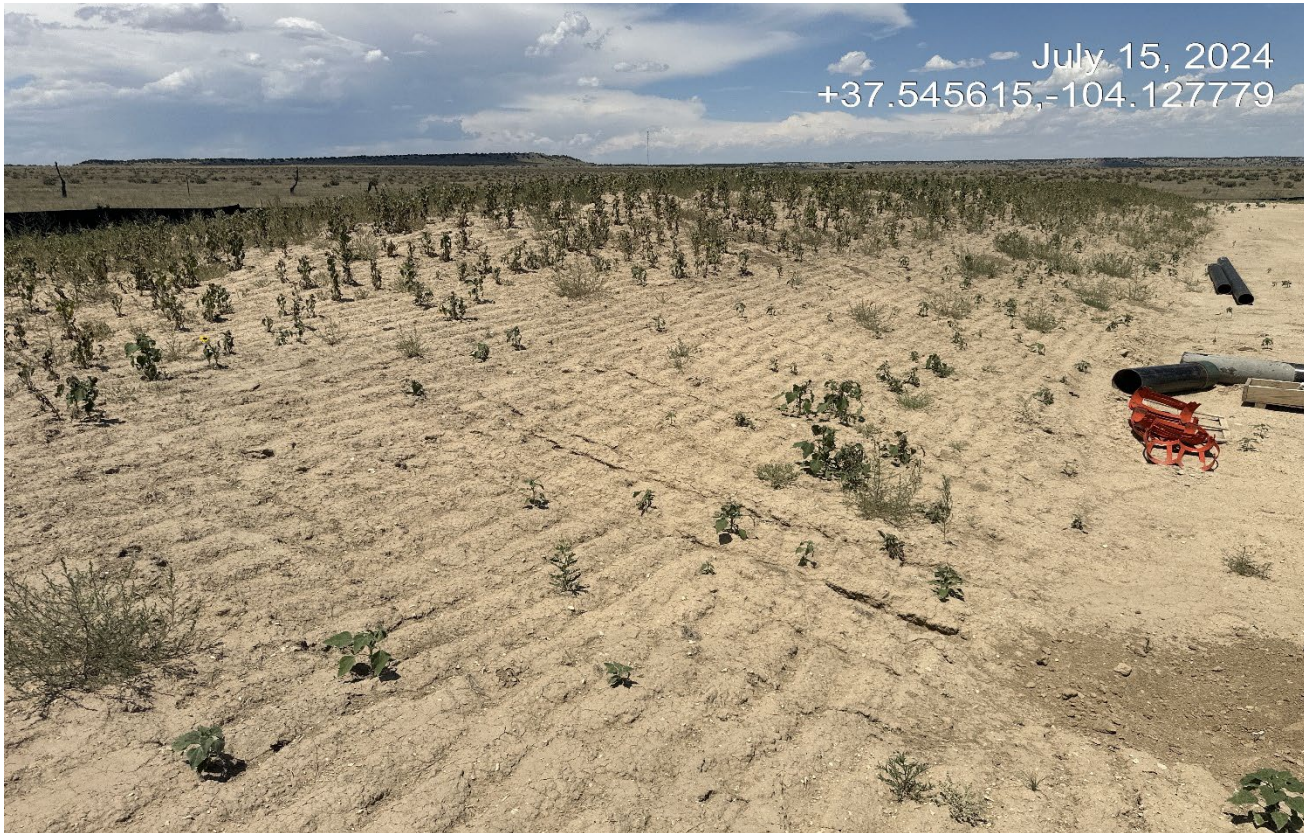
Photo 6. Facing toward the soil stock pile. The topsoil has not been seeded and stabilized and weeds are beginning to establish.
