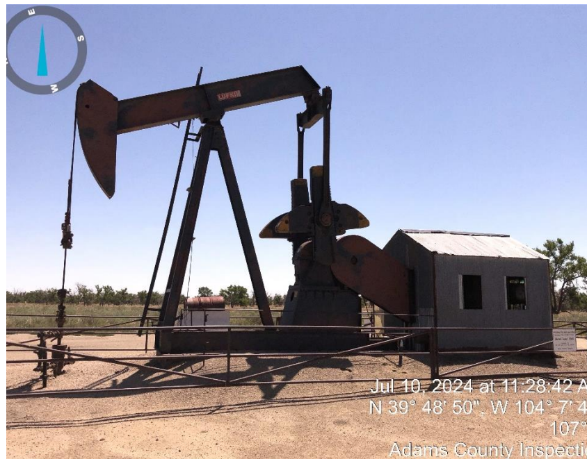
Photo #5 Pump jack.
