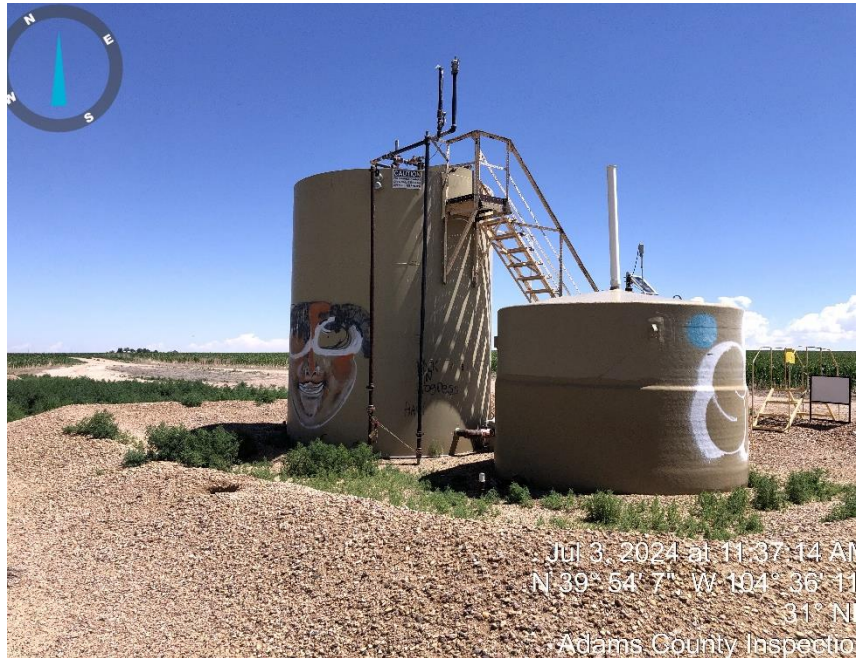
Photo #6 Weeds on and inside berm and Graffiti on crude and P/W tanks.
