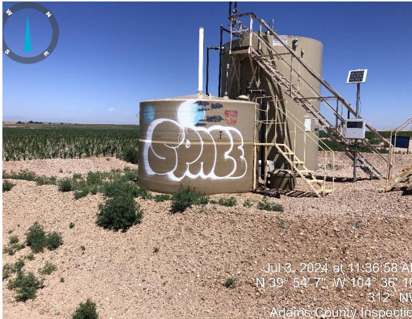
Photo #5 Weeds on and inside berm and Graffiti on P/W tank.
