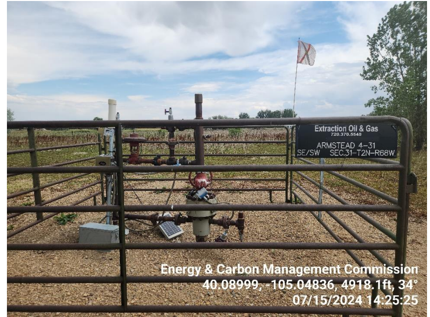
Photo 2 Wellhead & sign, SI LOTO
