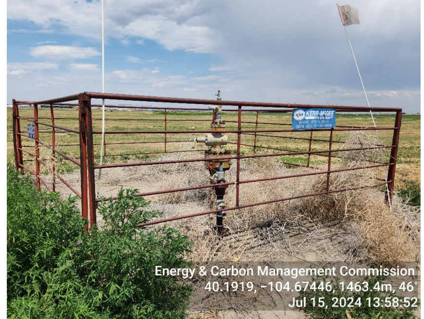
Photo 2: TA Wellhead, debris/overgrown vegetation
