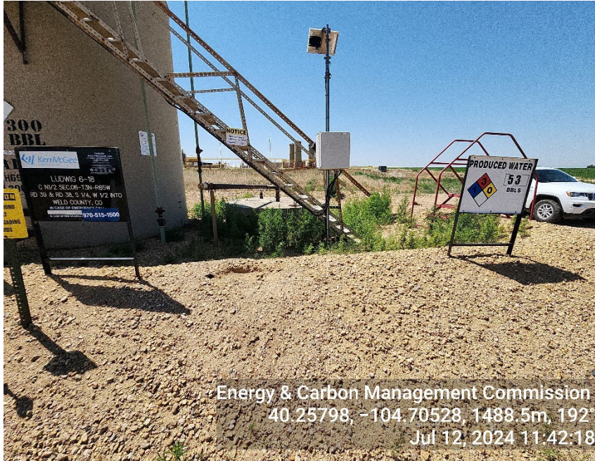
Photo 7: Weeds, holes in berm
