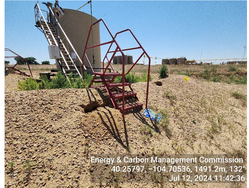
Photo 8: Weeds, holes in berm
