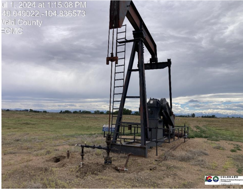
Pic 1 wellhead / pumpjack
