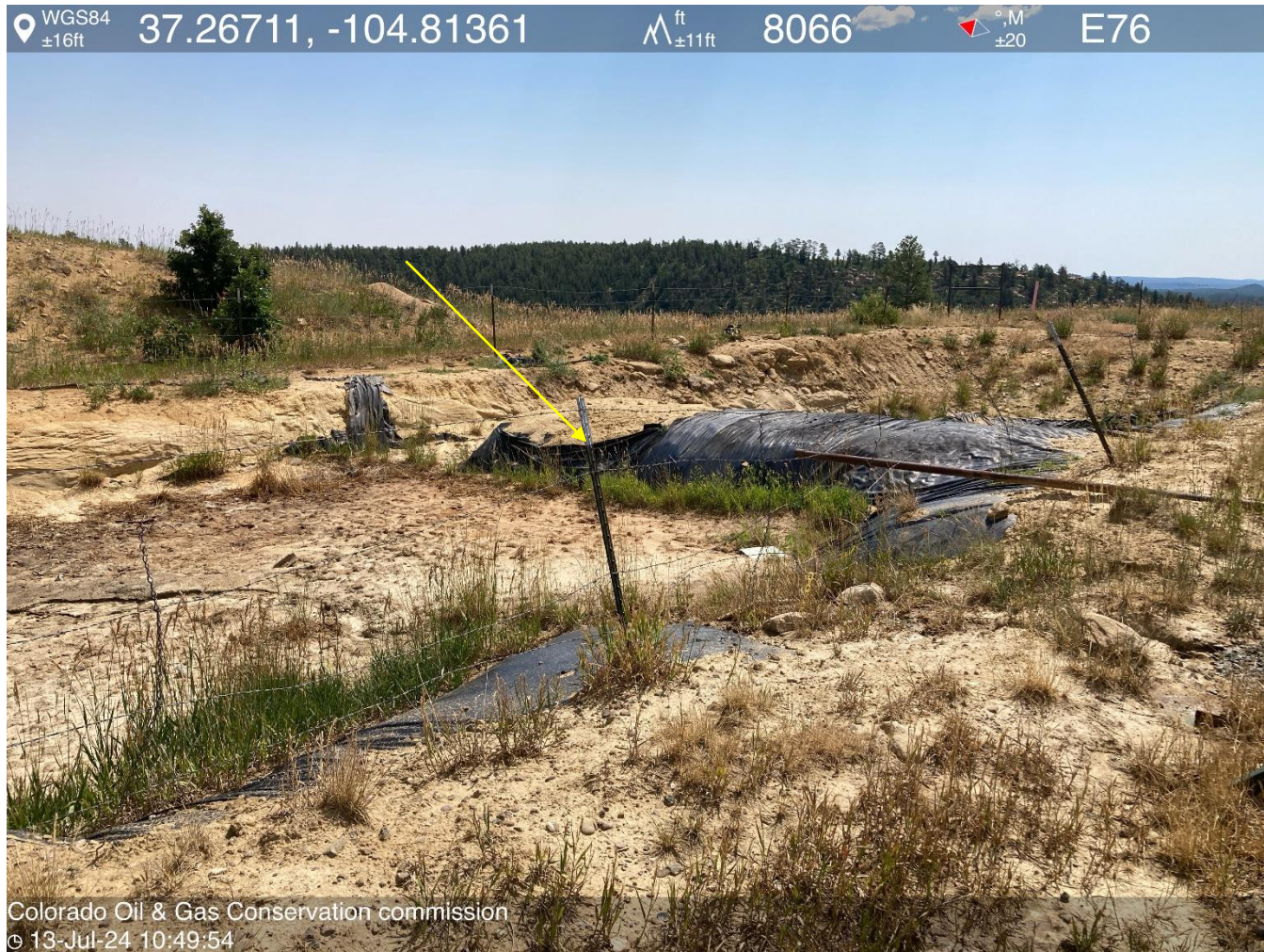
PHOTO 6: pit liner compromised. (Rule 910). contact COGCC EPS staff for directives. THIS IS THE SECOND NOTICE IMMEDIATE ACTION IS REQUIRED.
