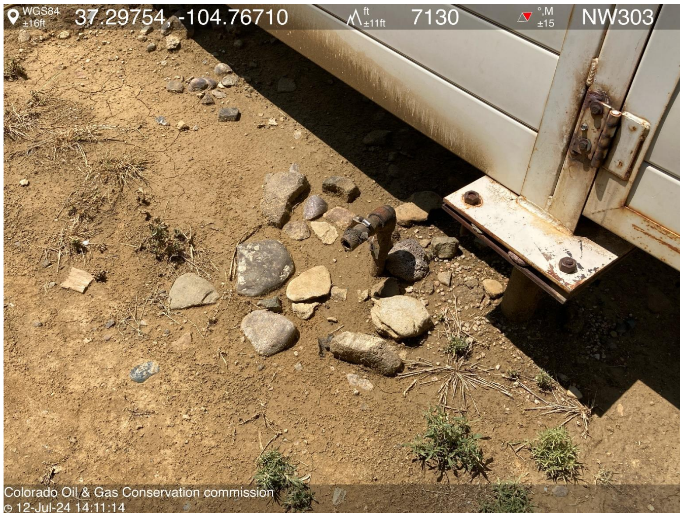
PHOTO 7: UNUSED EQUIPMENT (UNUSED 1" RISER NEAR COMPRESSOR SOUND WALLS). REMOVE OR MARK UNUSED RISERS PER RULE 606. CA DATE 8-12-2024.
