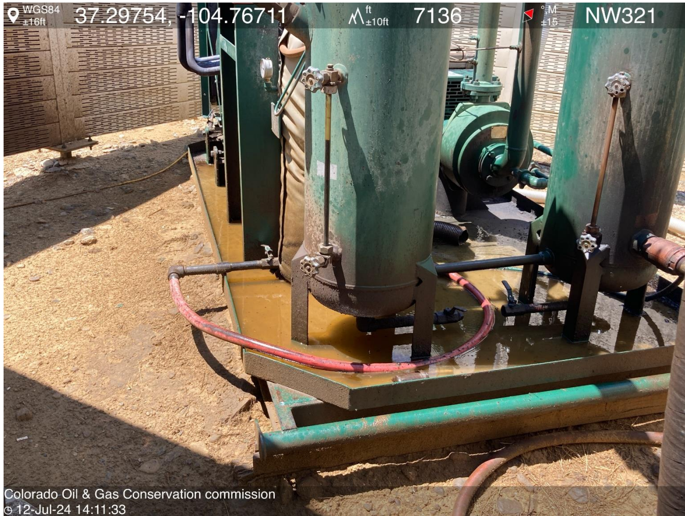
PHOTO 6: OILY WASTE IN COMPRESSOR SKID HAS SPILLED OVER CAUSING IMPACT SOIL SURROUNDING SKID. DRAIN OILY WASTE REPAIR ALL LEAKS AND REMOVE OR TREAT IMPACTED SOIL PER RULES 1002..(2).D & 1002.f.(2)B, Comply with general provisions of the oil and gas act for wildlife protection AND SB-181. CA DATE 7-13-2024.
