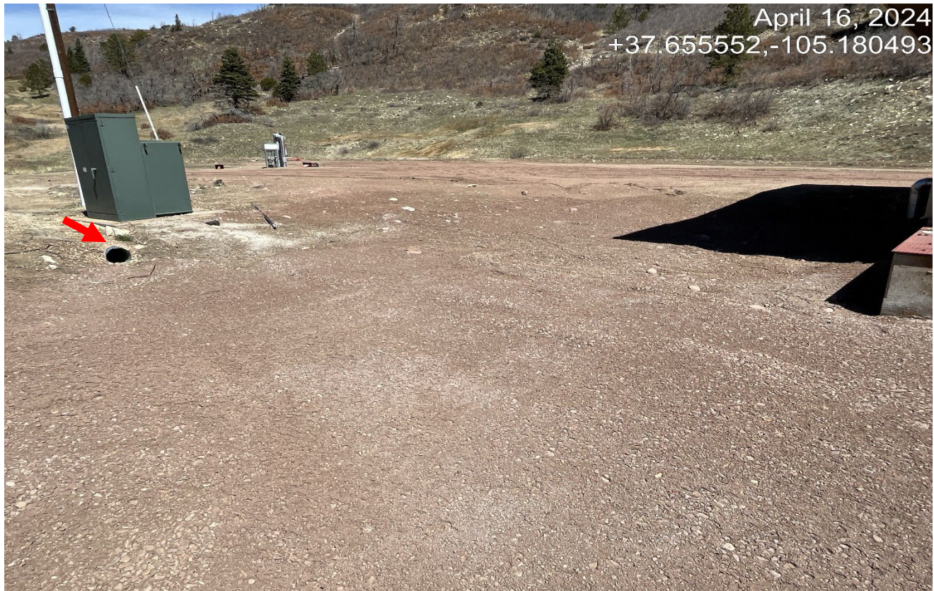
Photo 4. The remediation area where tank was located has been backfilled with sand and gravel. The red arrow points to a culvert that would allow a potential spill to flow all the way toward the southwest portion of the pad
