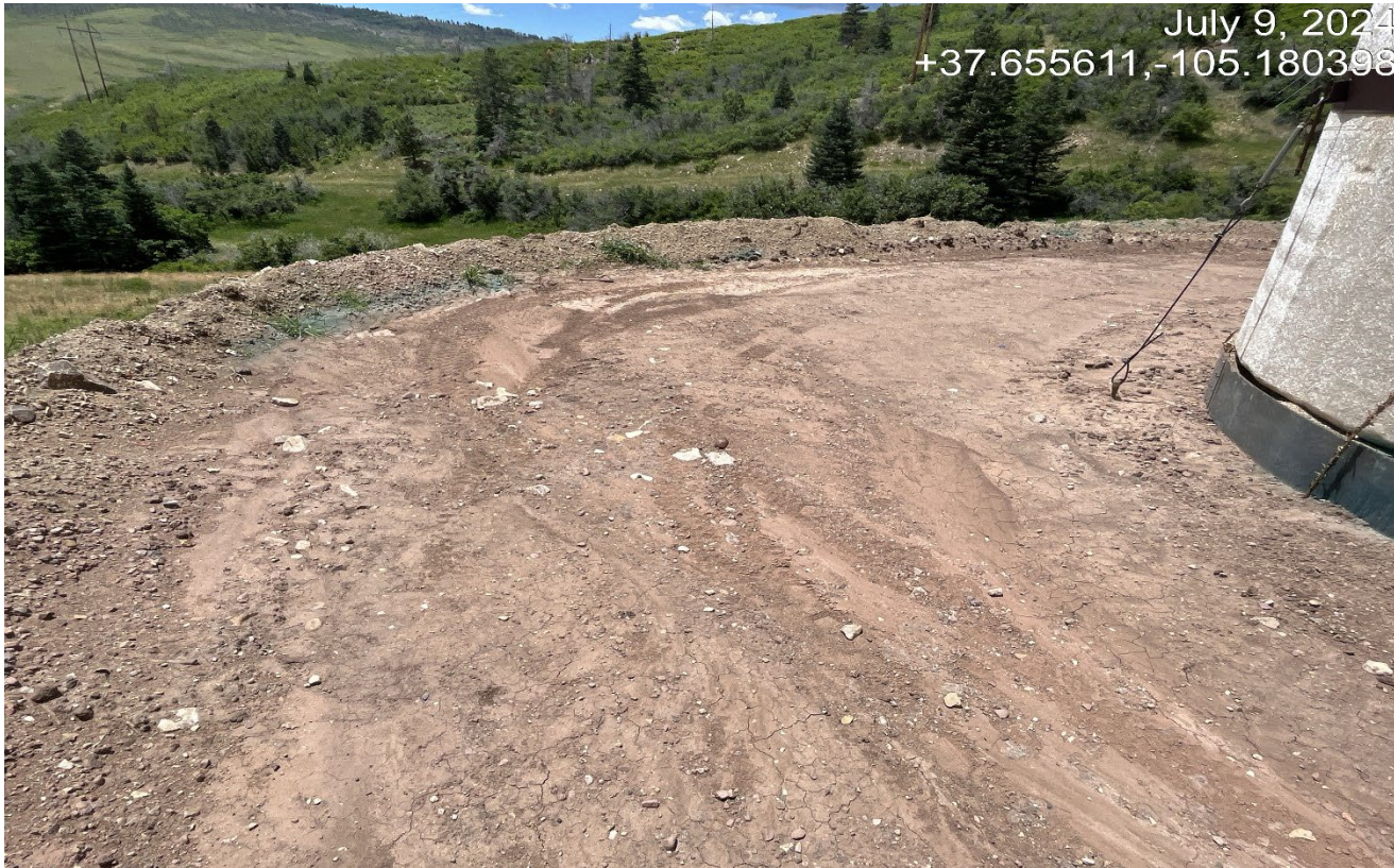
Photo 2. Facing toward the produced water tank. The secondary berm around the tank is insufficient to contain a spill. Previous corrective action was not completed.
