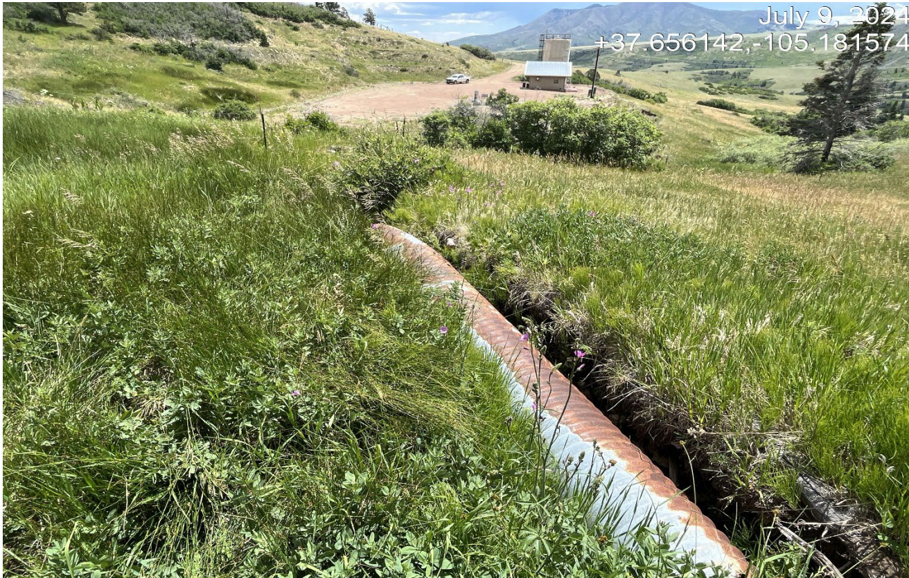
Photo 9. Standing approximately 125' west of the location along the flowline area is an eroded out culvert where the creek flows. The culvert needs repaired or removed. Previous corrective action was not completed.
