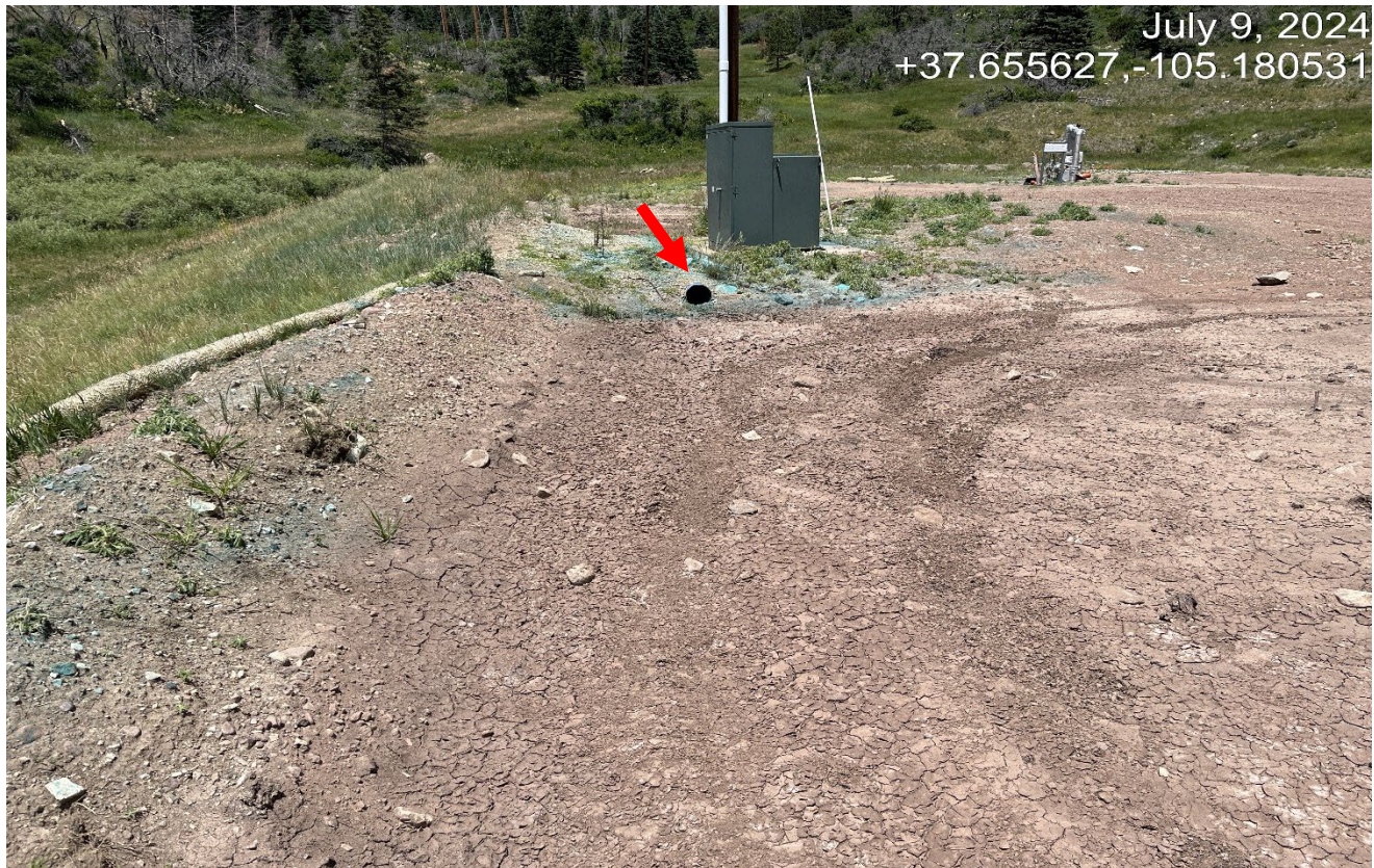
Photo 5. Wattles were installed along the southeast side but stop at this point. The red arrow points to a culvert that would allow a potential spill to flow all the way toward the southwest portion of the pad.
