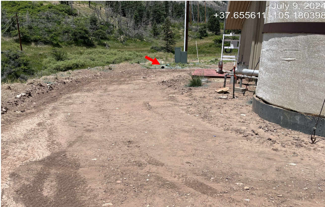
Photo 3. Facing west at the backside of the tank. The secondary containment at the tank is insufficient to contain a spill. The red arrow points to a culvert that would allow a potential spill to flow all the way toward the southwest portion of the pad near the perennial stream.
