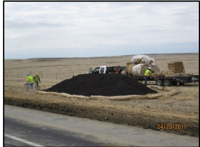
Erosion Logs used for stockpile management practices
