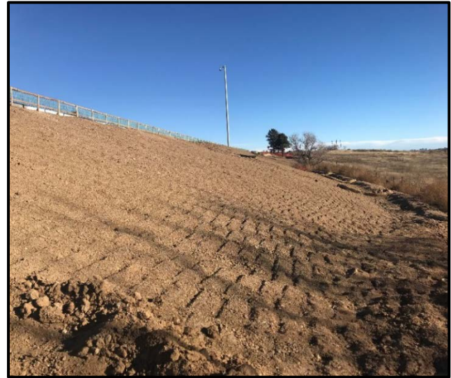
Vertical tracking on disturbed side slope
