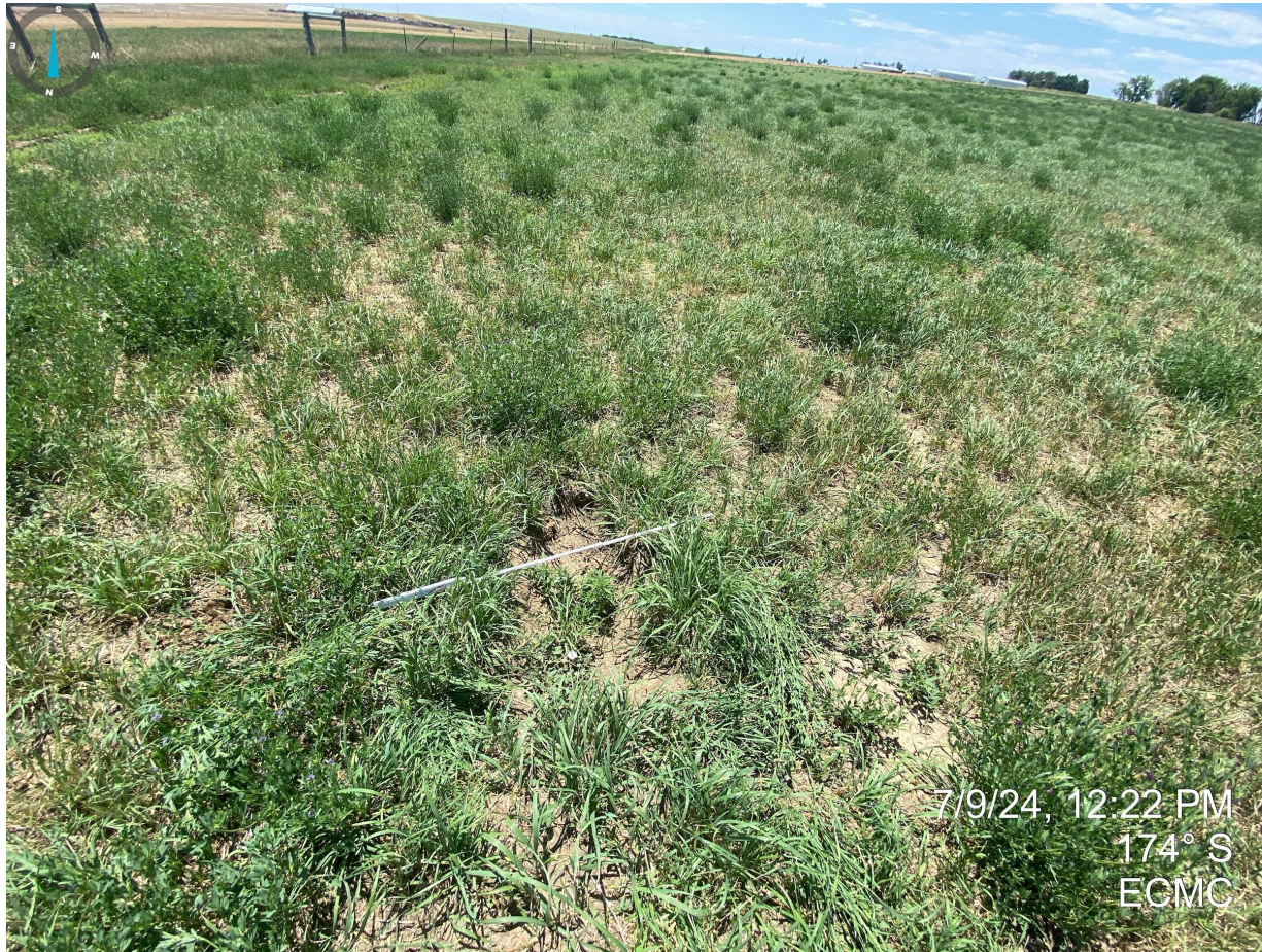
Photo 8. Subsidence observed at one of the flowline potholes.
