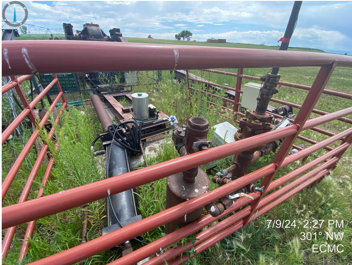
Photo 2. Pump jack is disassembled.
