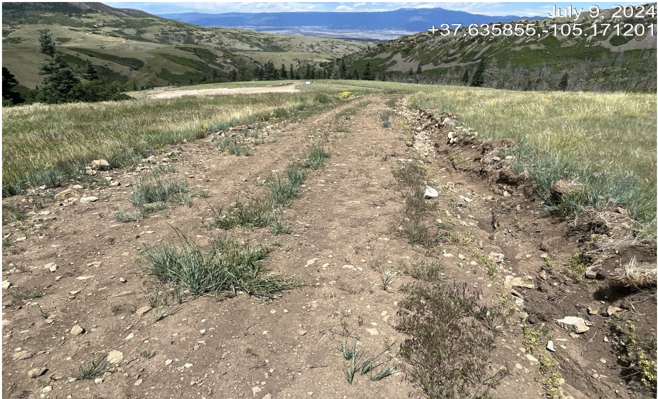
Photo 3. Facing northeast back down the access road. There are no BMP's to control erosion along this entire stretch of road
