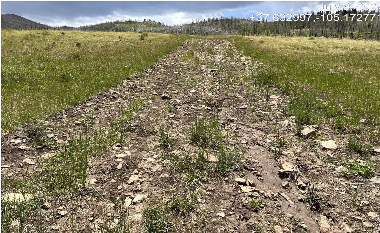
Photo 5. Facing southwest further along the access road. There is more vegetation establishment but there is still erosion along the road. Stormwater should be diverted off the road.
