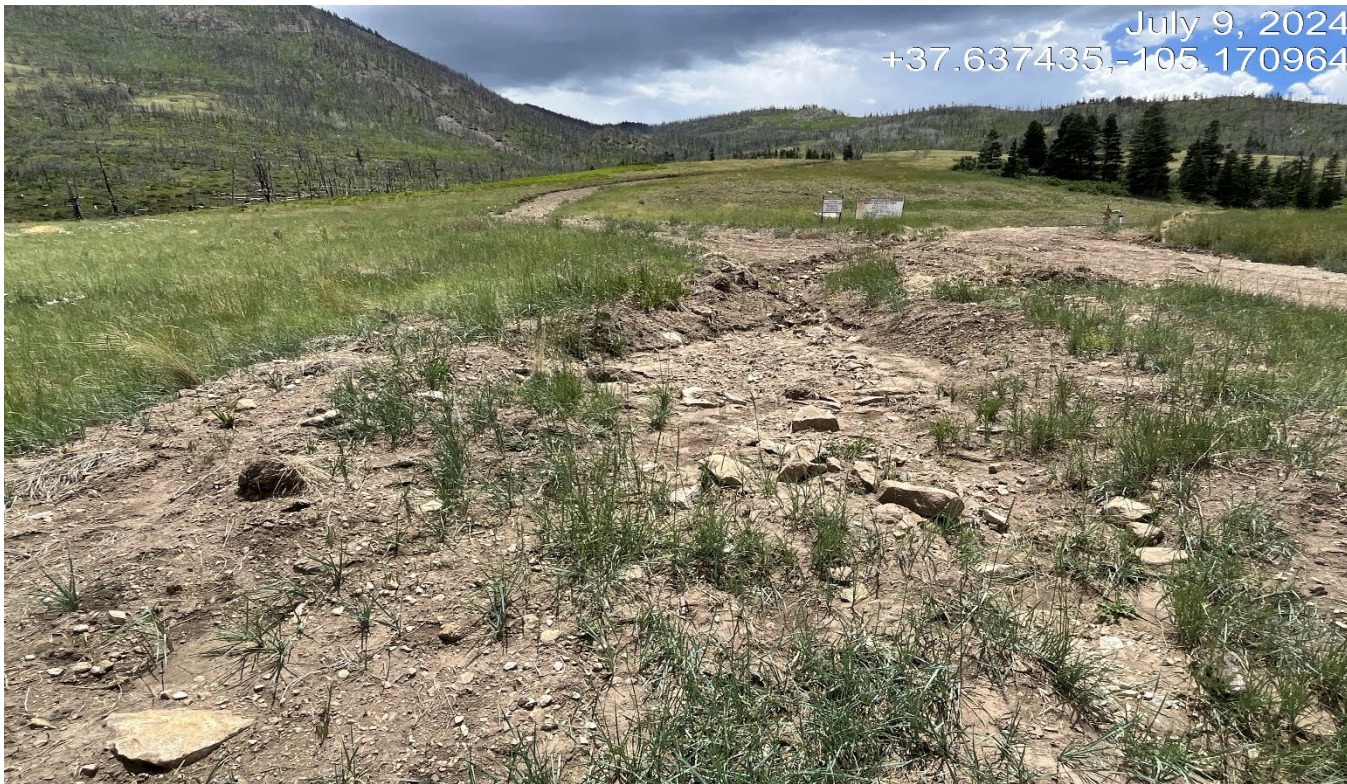
Photo 1. Facing southwest along the access road near the SMU #1-12-B . Sediment has been deposited and pushed off the road into this area creating additional disturbance.
