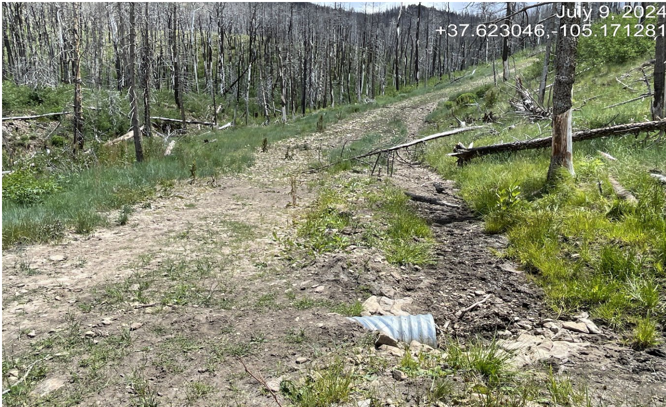
Photo 6. Facing southwest further along the access road. This culvert has filled in with sediment.
