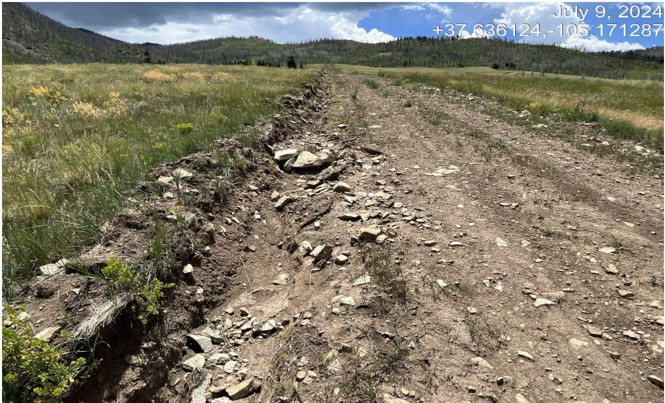
Photo 4. Facing southwest along the access road. There is erosion that has occurred along the road which has no BMP's to control erosion.
