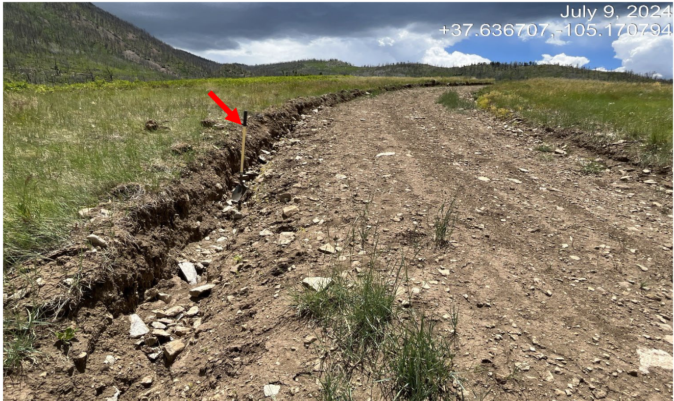
Photo 2. Facing southwest along the access road. There is erosion that has occurred along the road. Red arrow points to shovel placed in the erosion channel.
