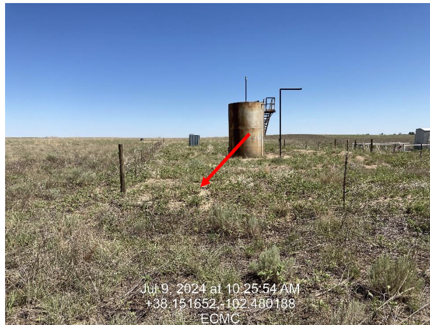
Photo 4 – Tank Battery fencing not adequately maintained
