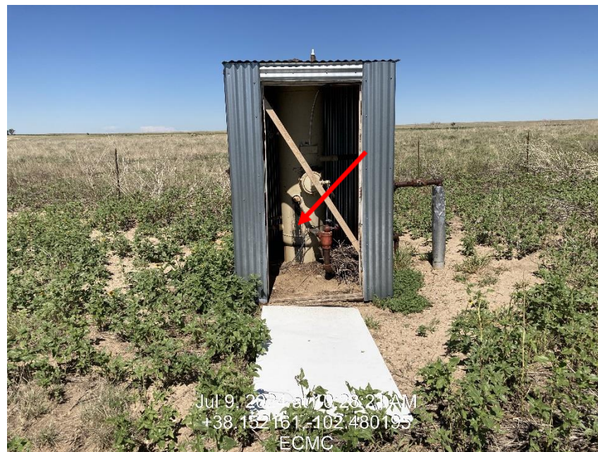
Photo 8 – Door to separator house not attached to building
