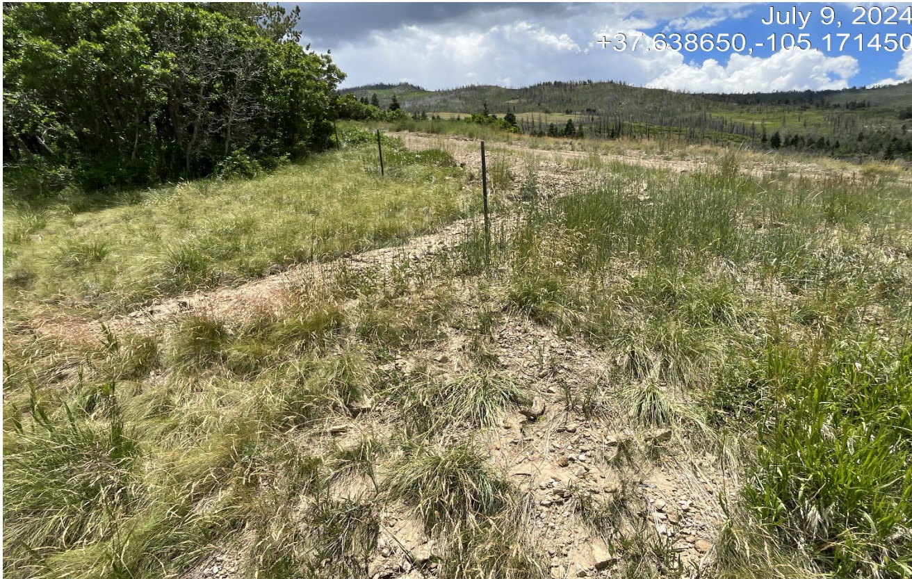
Photo 3. There is sediment that has been transported offsite along the road. A BMP such as a sediment trap should be installed to control erosion.
