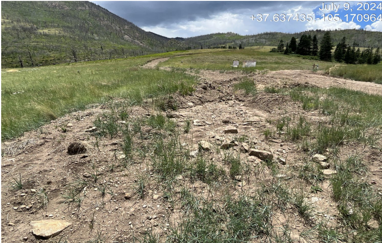
Photo 6. Facing southwest along the access road near the SMU #1-12-B . Sediment has been deposited and pushed off the road into this area creating additional disturbance.
