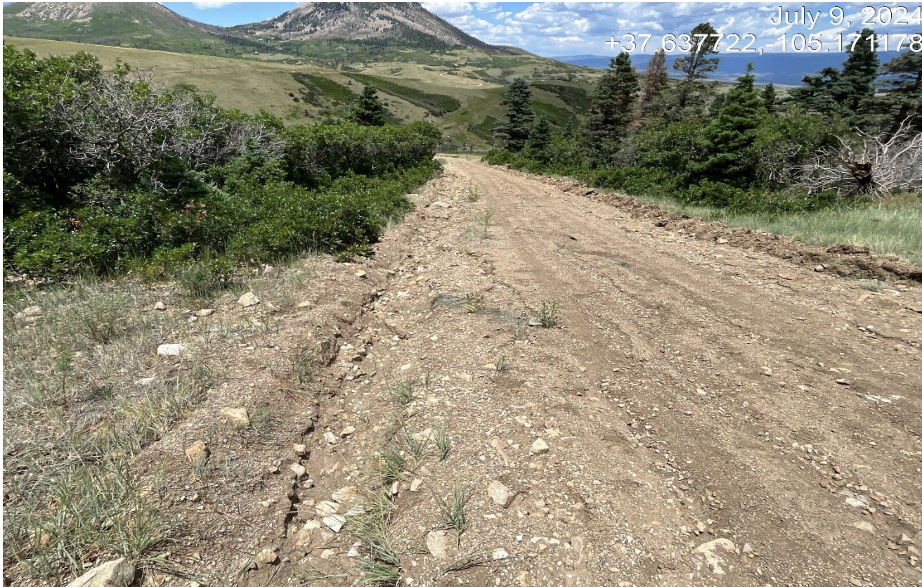
Photo 5. Facing north along the steep grade of access road. Stormwater is directed all the way down this road and there are no BMP's for sediment control.
