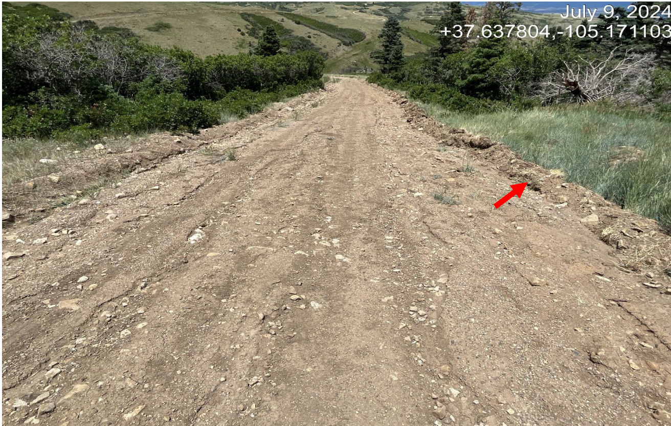
Photo 4. Facing back north the steep grade of access road. Stormwater is not being diverted off the road which is causing erosion of the road. Stormwater should be divert toward red arrow and into a sediment trap.
