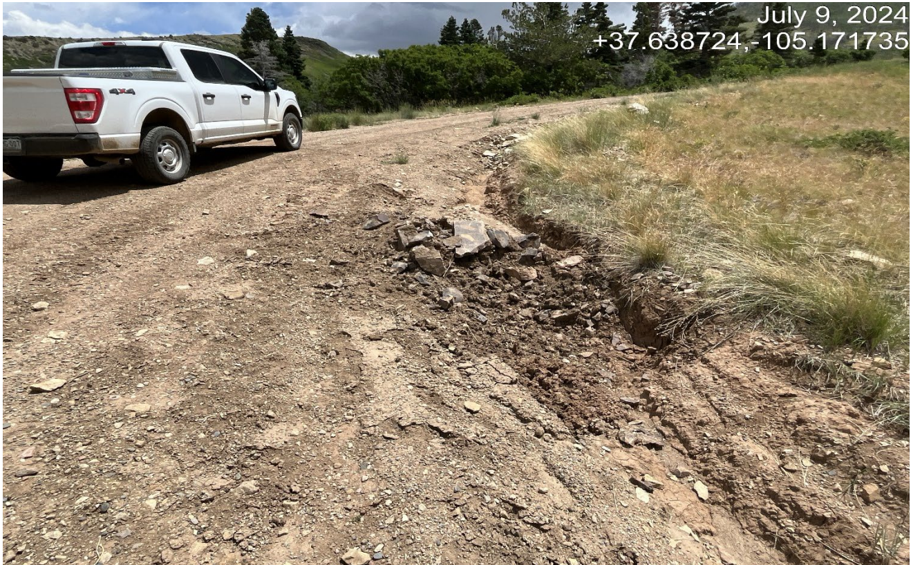
Photo 2. Facing southeast along the access road. There is rock and soil pushed up along the road side. This is not an adequate stormwater control.
