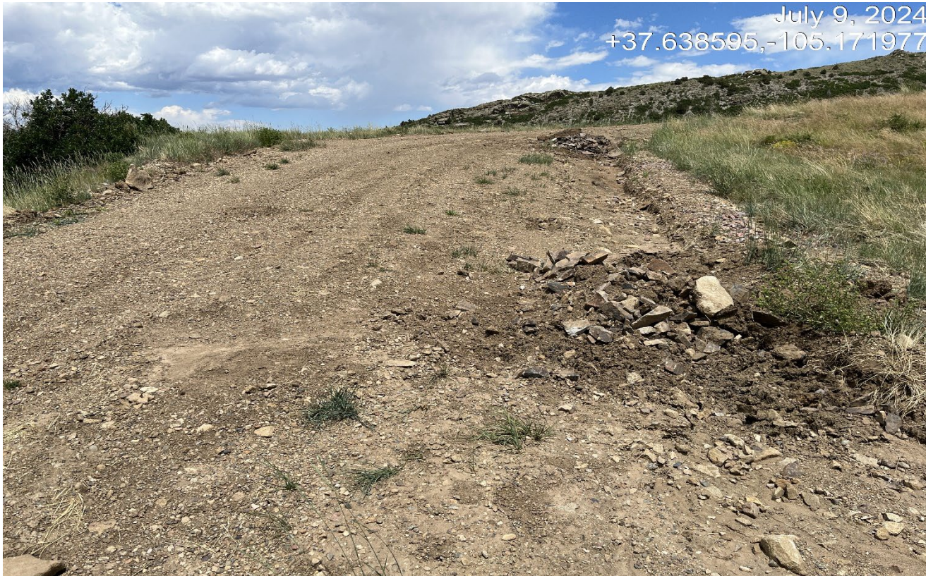
Photo 1. Facing east along the access road. There is rock and soil pushed up along the road side. This is not an adequate stormwater control.
