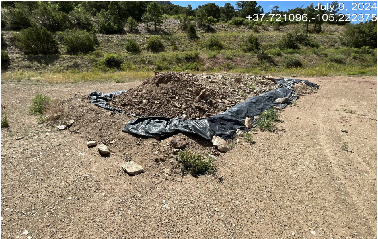
Photo 5. The plastic liner is compromised and impacted soil needs to be removed.
