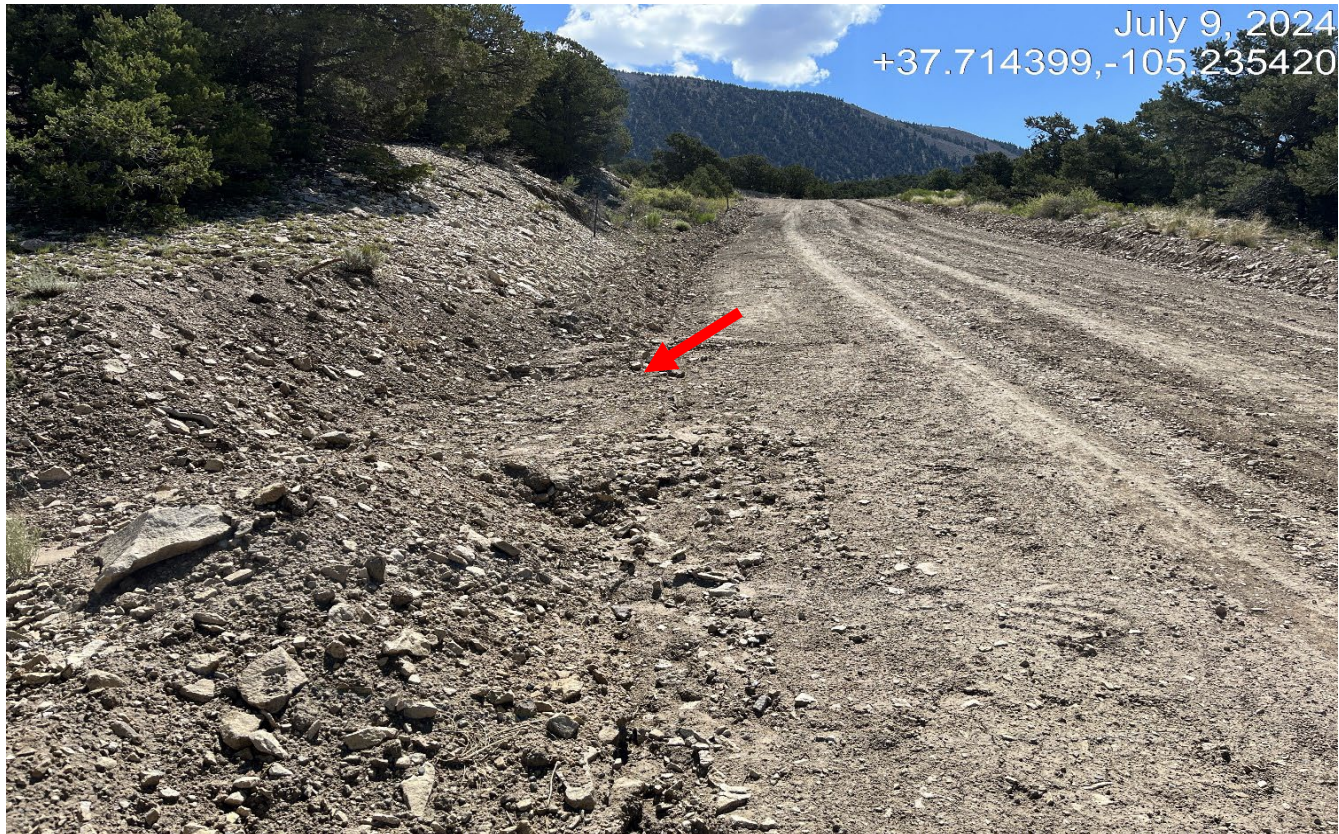
Photo 1. Facing east along the access road. Grading has been performed to allow drainage off the road.
