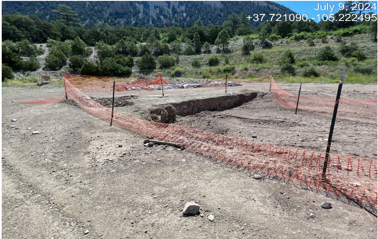
Photo 4. Facing toward the abandoned wellhead which has been backfilled with road base material.
