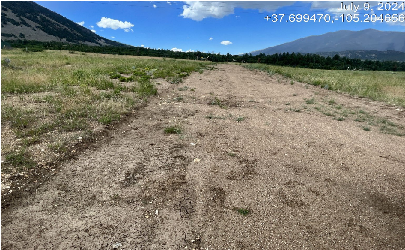
Photo 1. Facing south toward the access road.. The access road will need to be decompacted and reclaimed. Previous corrective action has not been completed.
