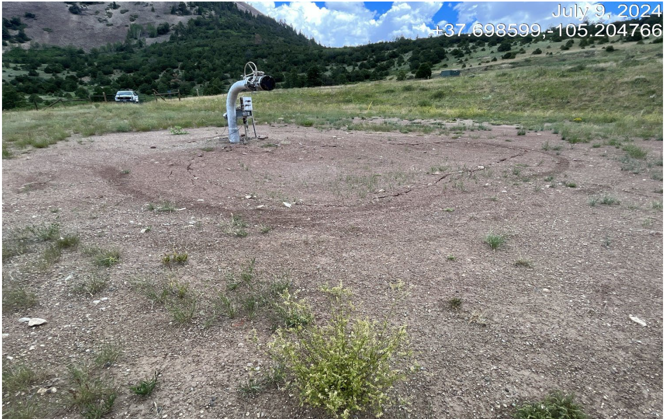
Photo 6. Facing toward the abandoned well which was cut and capped. The remaining pipe riser must be removed.
