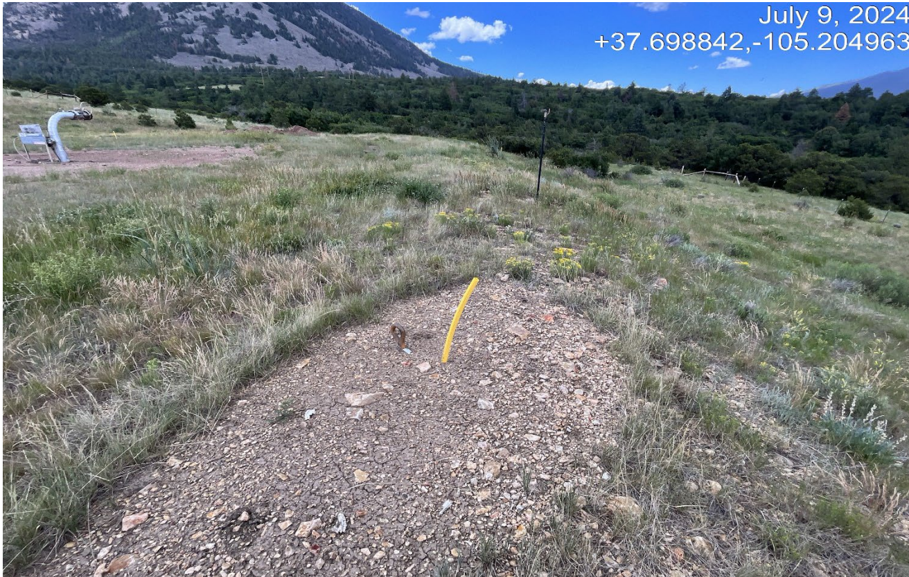
Photo 4. Facing south toward the fill slope which must be recontoured back to the original condition. The four guyline anchors need to be removed along with the pipe riser shown in this photo.
