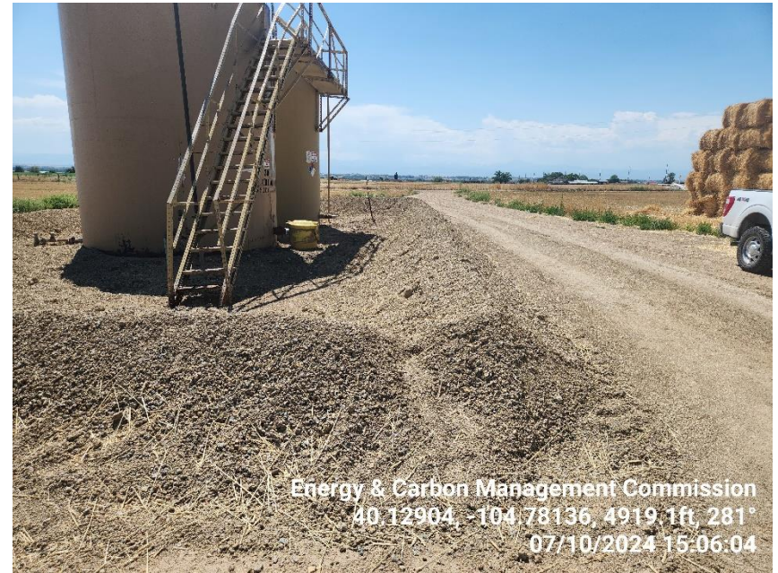
Photo 8 Unlined gravel berm around the tank battery not in compliance with Rule 603.o.
