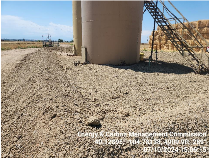
Photo 9 Unlined gravel berm around the tank battery not in compliance with Rule 603.o.
