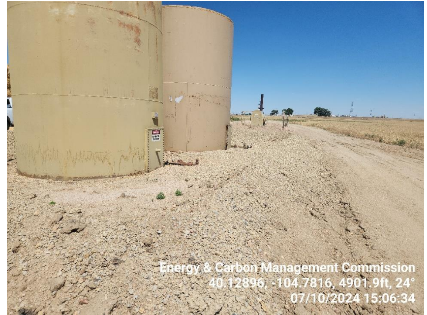
Photo 10 Unlined gravel berm around the tank battery not in compliance with Rule 603.o.
