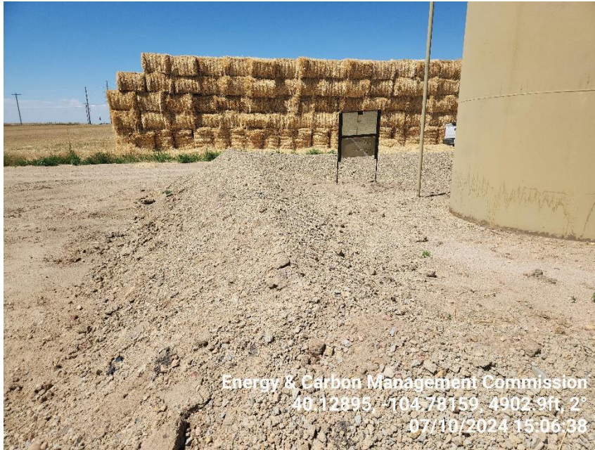
Photo 11 Unlined gravel berm around the tank battery not in compliance with Rule 603.o.
