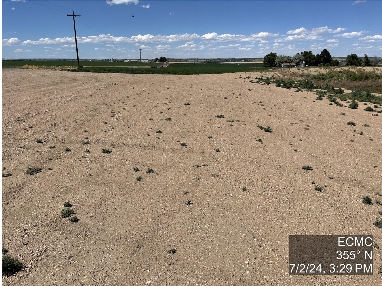
Photo 7. The photo was taken at the tank battery location. The photo illustrates the former tank battery location is stabilized with compact road base.
