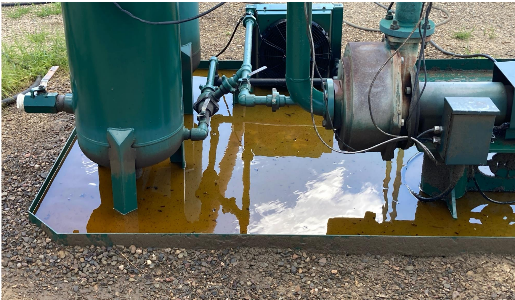
PHOTO 4: OILY WASTE FROM LEAK IN HYDRAULIC MOTOR HAS FILLED SKID AND HAS SPILLED OVER CAUSING IMPACT SOIL SURROUNDING SKID. DRAIN OILY WASTE REPAIR ALL LEAKS AND REMOVE OR TREAT IMPACTED SOIL PER RULE 1002.f.(2)B, Comply with general provisions of the oil and gas act for wildlife protection AND SB-181.
