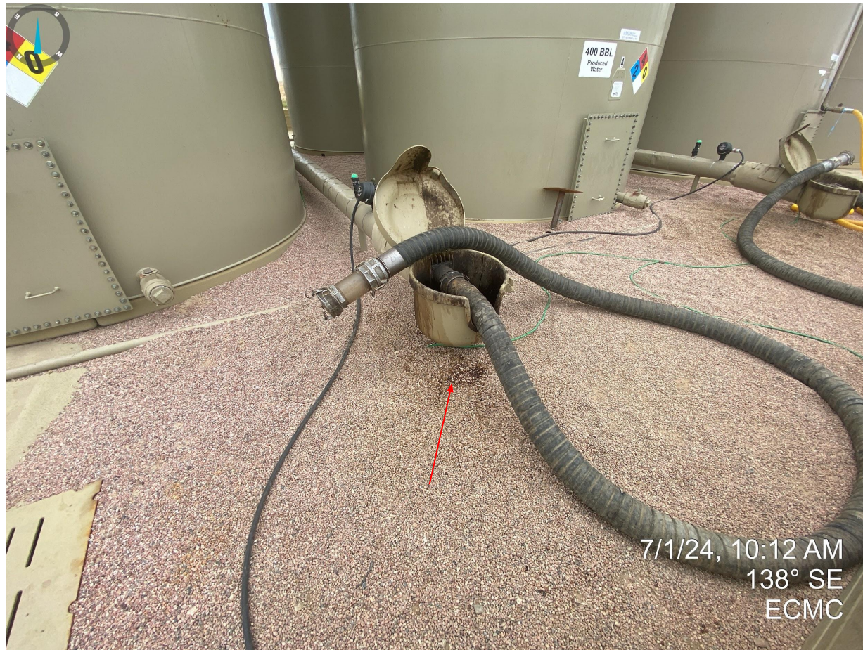
Photo 21. Stained soil within tank battery secondary containment.
