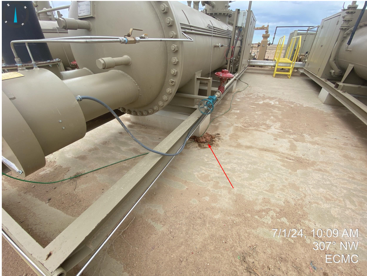
Photo 16. Staining and debris observed within secondary containment at separator.
