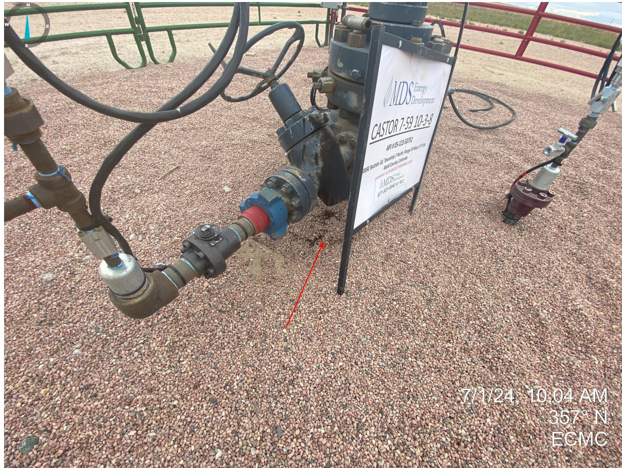
Photo 13. Stained soil observed near wellhead.
