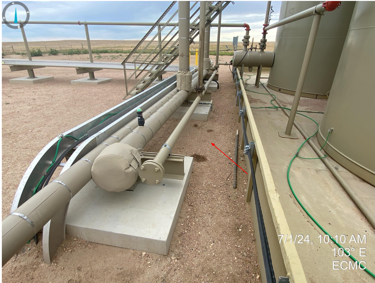
Photo 18. Stained soils observed on north end of tank battery.
