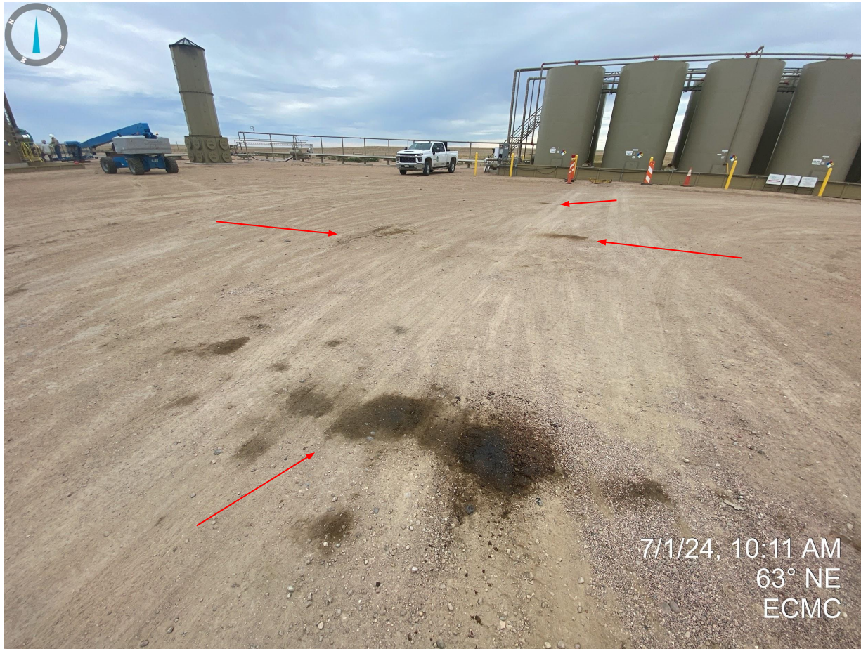
Photo 19. Stained soils observed west of tank battery.
