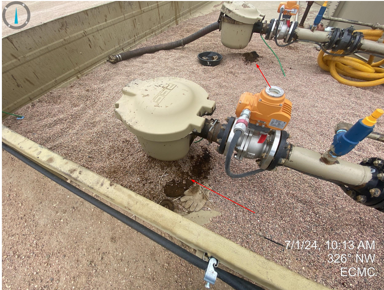
Photo 24. Stained soil within tank battery secondary containment.
