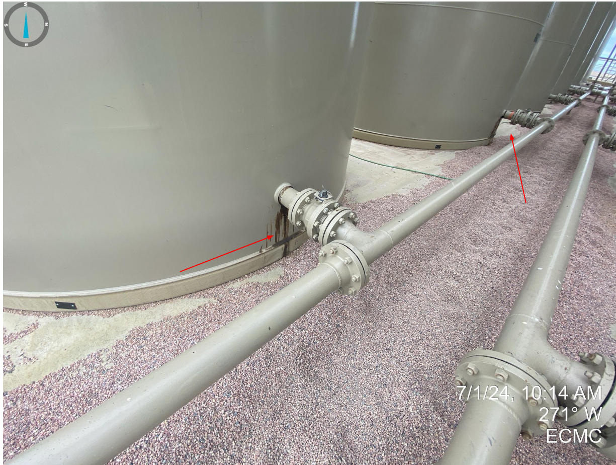
Photo 25. Leaking equipment requires maintenance.
