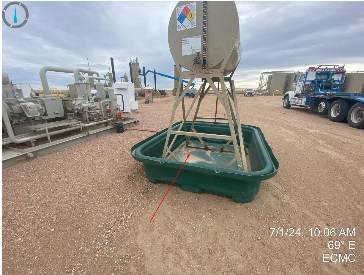
Photo 15. No wildlife netting observed at secondary containment.
