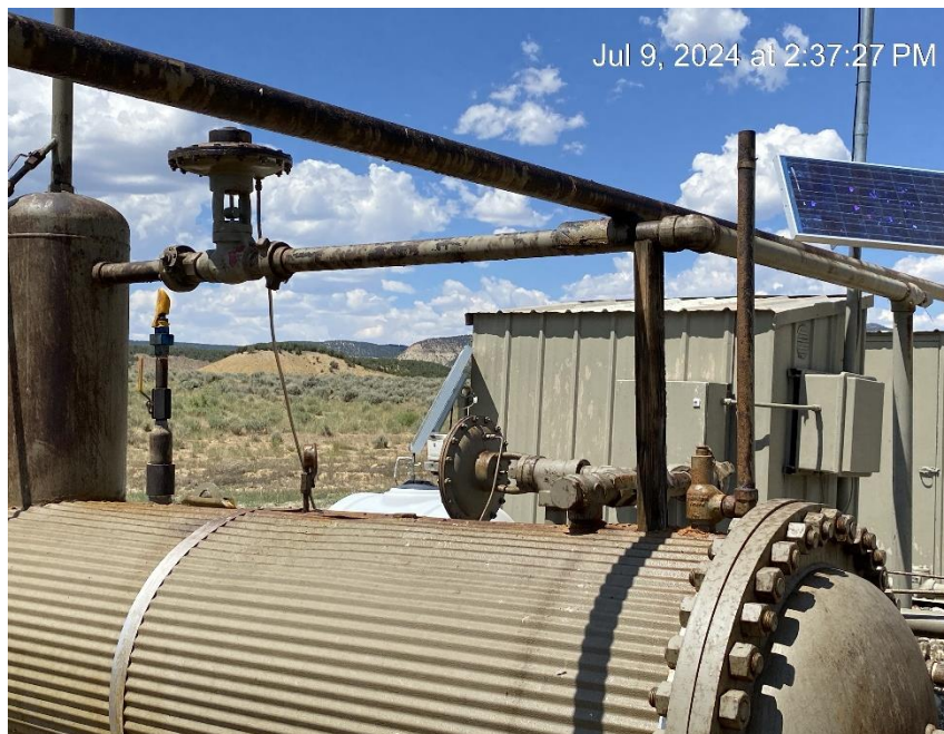
Relief riser missing protective cap
