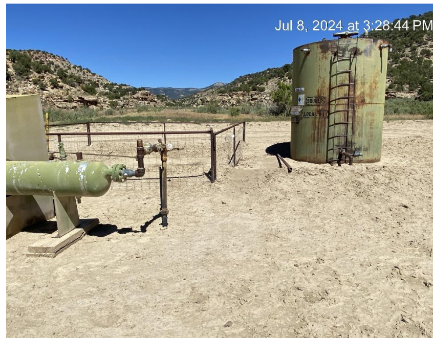
Berm capacity inadequate
