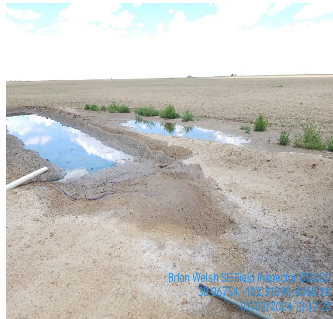
4. Standing inside the berms looking north. Spill had breached the berms and went outside of containment
