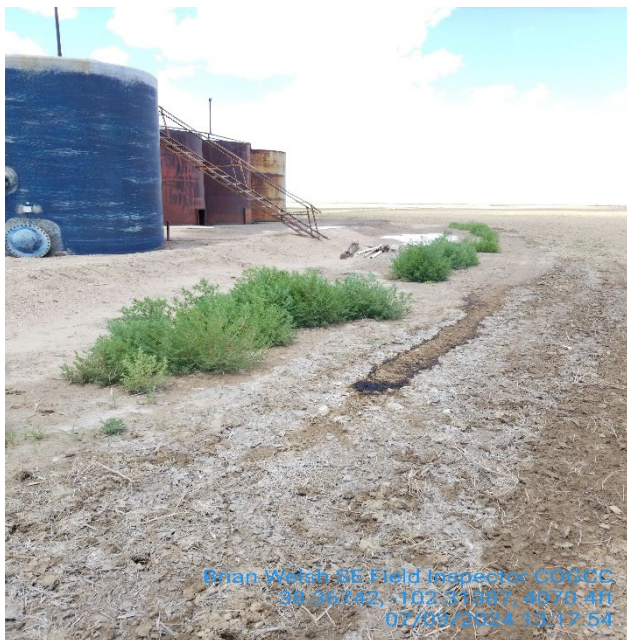
3. Southeast corner of tank battery looking north at spill outside of berms. There is some crude oil from the spill that traveled south in the adjacent cropland
