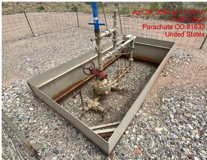
Open Wellhead Cellar – Photo #02118
