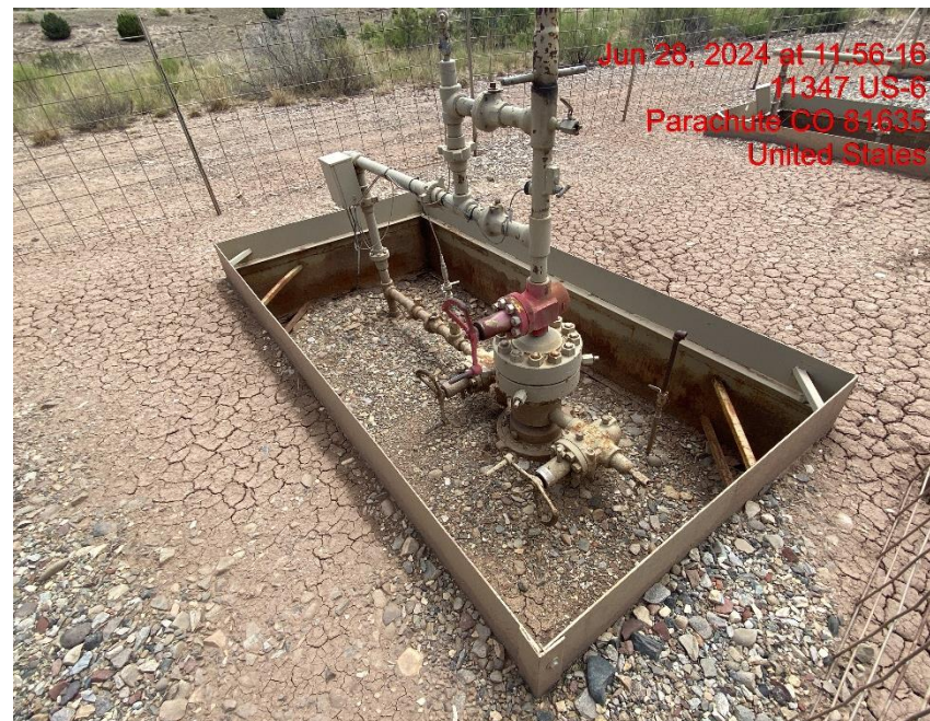
Open Wellhead Cellar – Photo #02119
