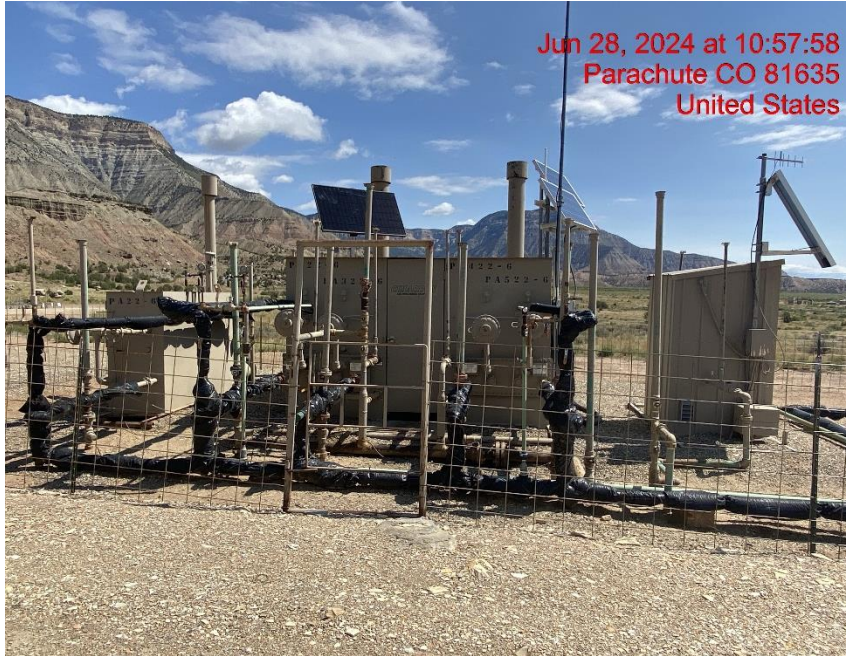
Separators/Gas Meter – Photo #02087
