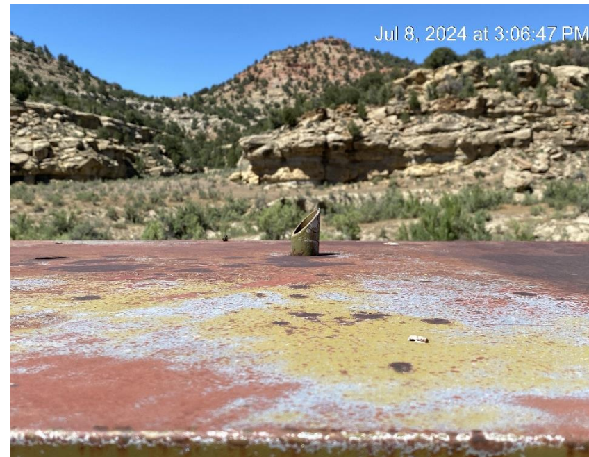
Relief riser missing cap
