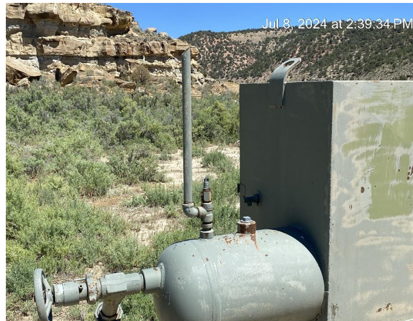
Relief riser protective cap missing
