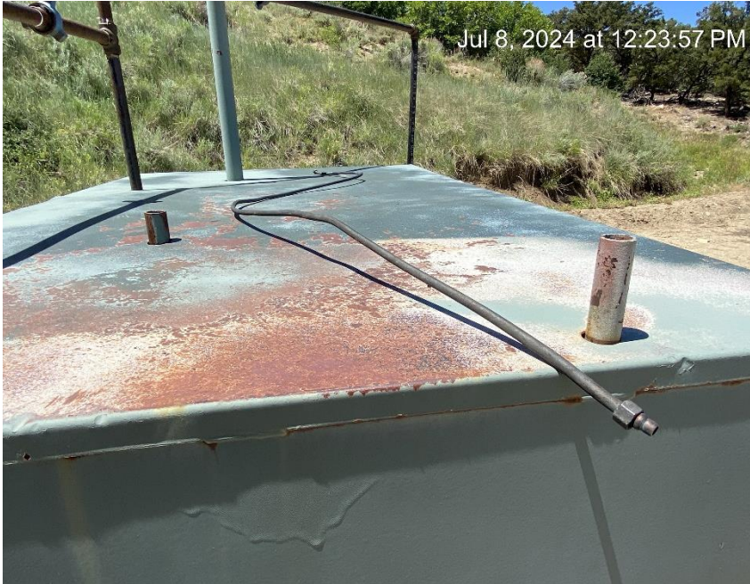
Debris. Relief riser cap missing.
