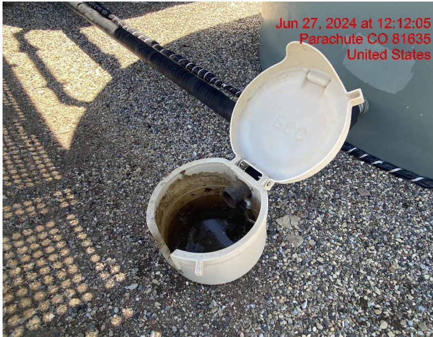
Open-Ended Load Line – Photo #02048
