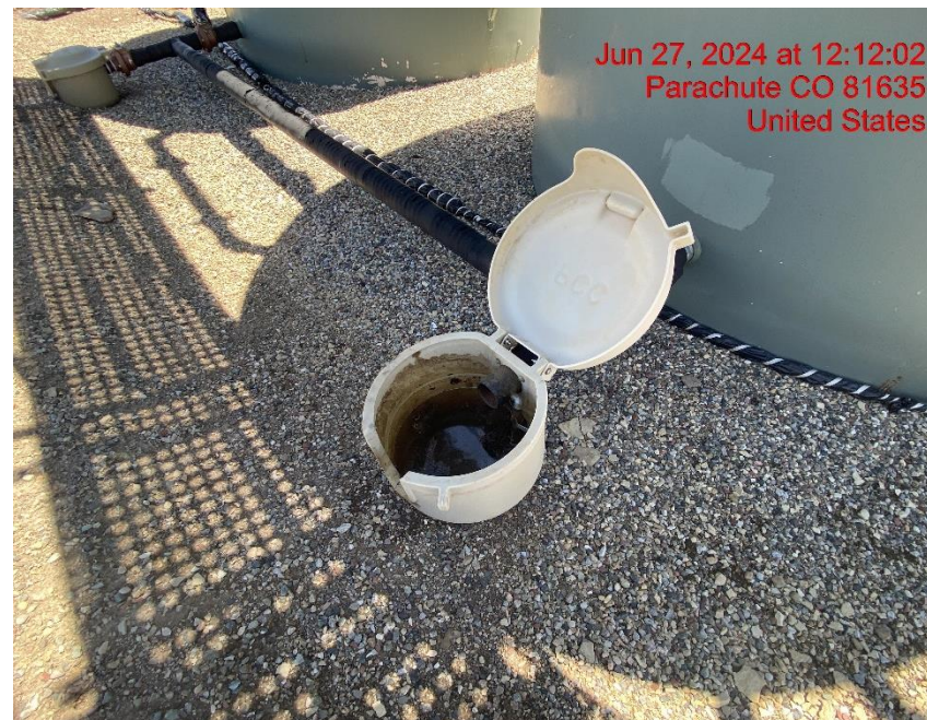
Open-Ended Load Line – Photo #02047
