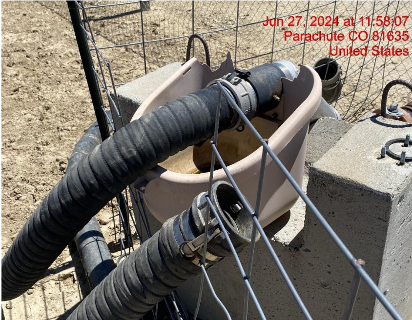
Open-Ended Offload Line – Photo #02019
