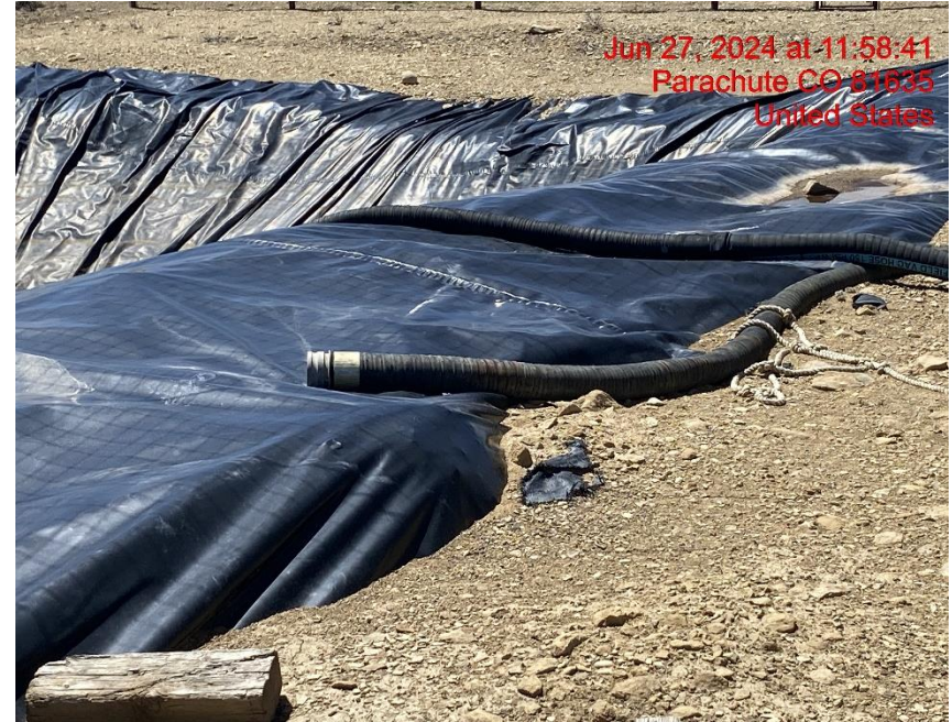
Open-Ended Offload Line into Pit – Photo #02022
