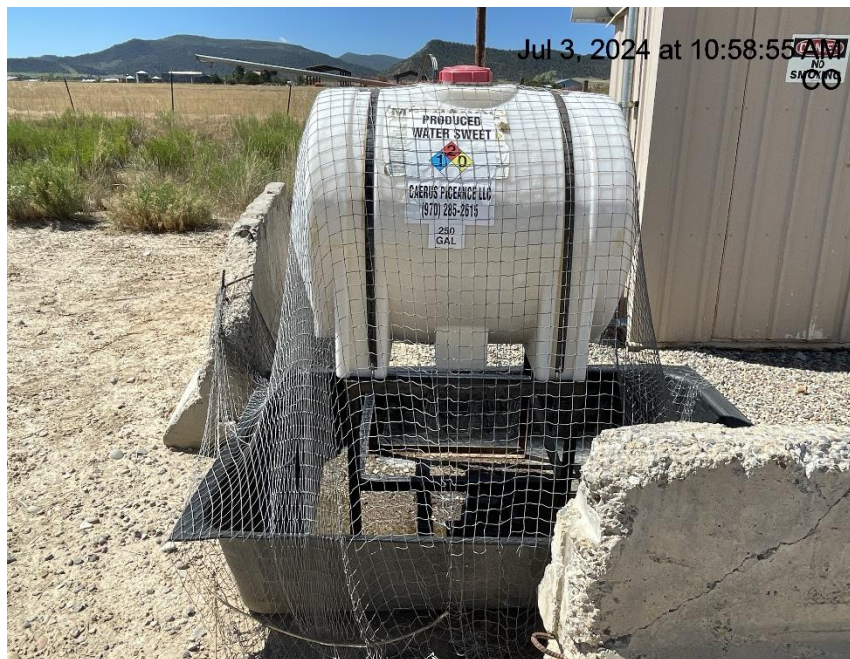
Photo # 2425 Chemical tank is in use/used for water sampling/monitoring due to previous spill - please refer to FORM 4 SUNDRY document # 403739635
