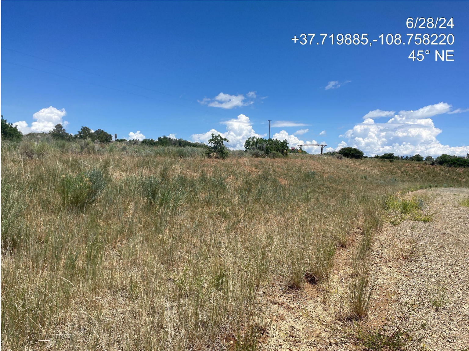
Photo 2. View of project area cut slopes that have been reduced to a slope of 3:1 and are revegetated with desirable vegetation to the 80% vegetation standard.
