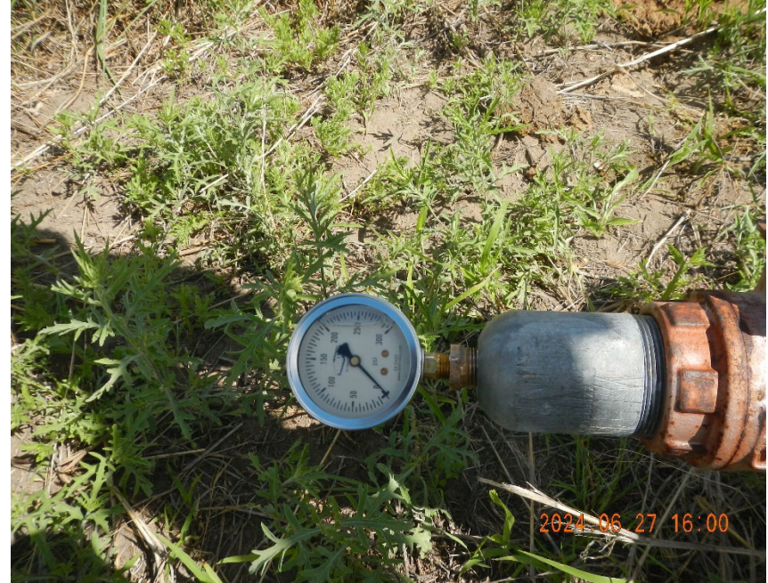
4. Casing pressure at time of inspection.
