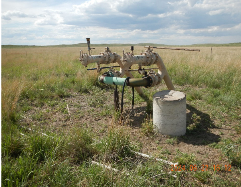
11. View of one of the Pig Stations. Stock Panels are down lying on the ground. Cattle tracks around station.
