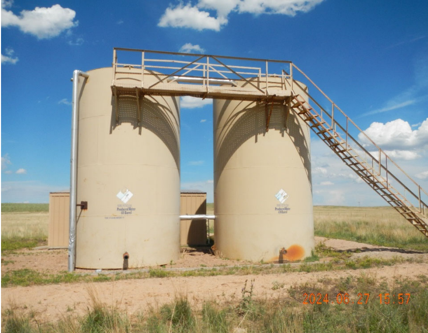
9. View of Steel AST's. Note rust at valve area on right tank.
