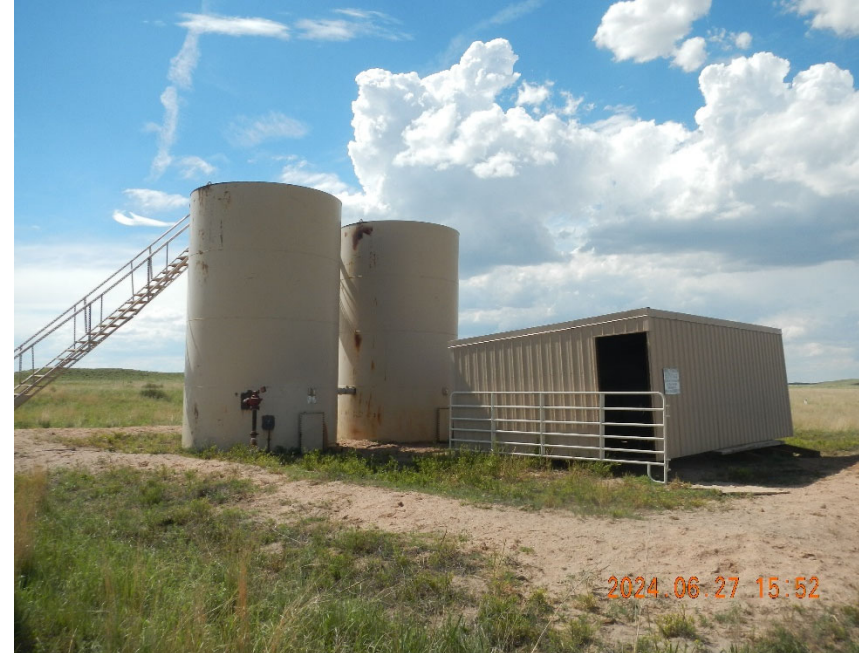
6. View of Tank Battery. Note vegetation inside berms and berms flatness due to wear.
