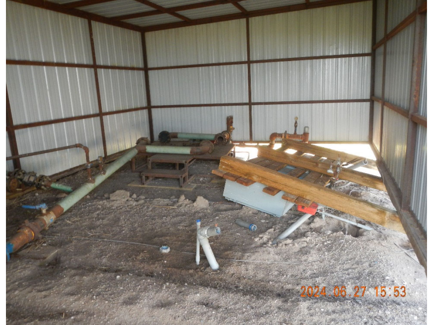
8. Inside metal shed. Trash, debris, unused equipment, open ended flowlines, and broken off panel supports.
