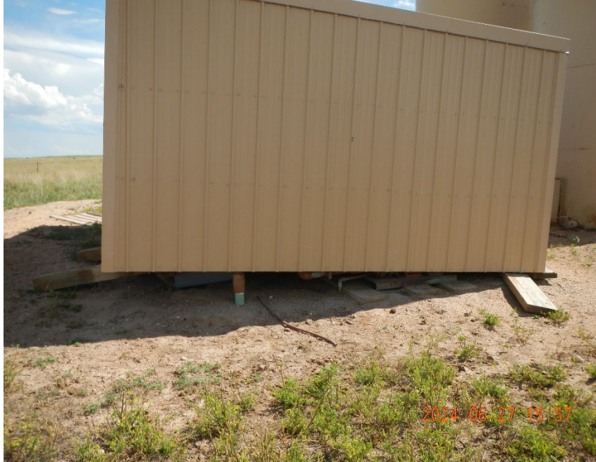
7. Metal building leaning and off footings.
