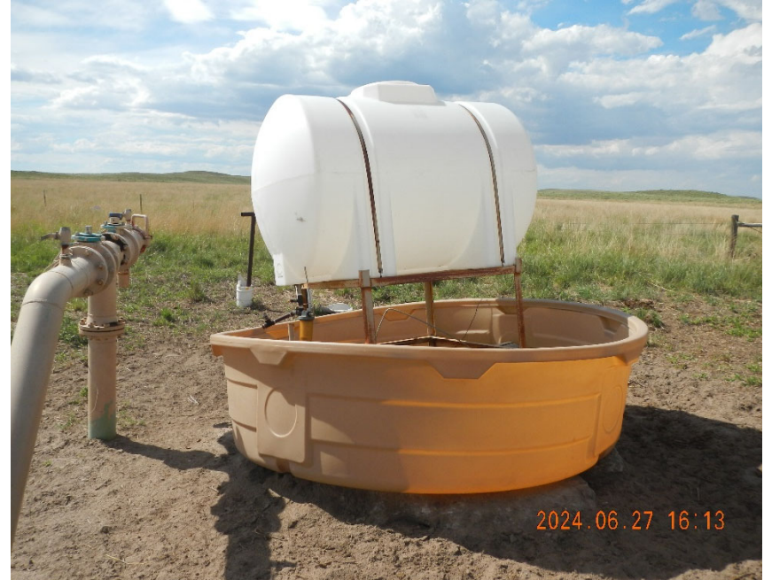
12. Chemical Tank inside secondary containment. Located at Pig Station. Tank has no labels.
