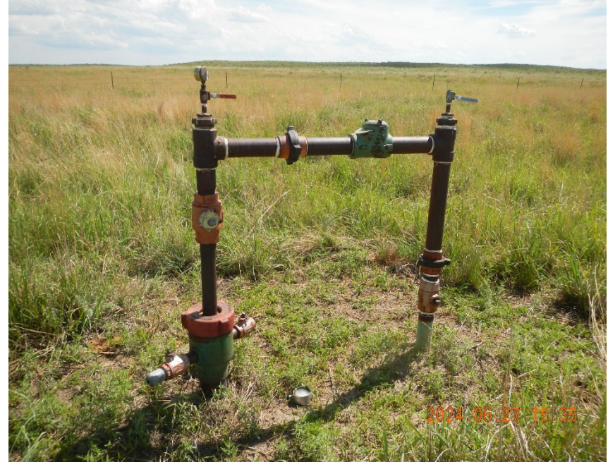
2. View of wellhead. Note missing Bull plugs.
