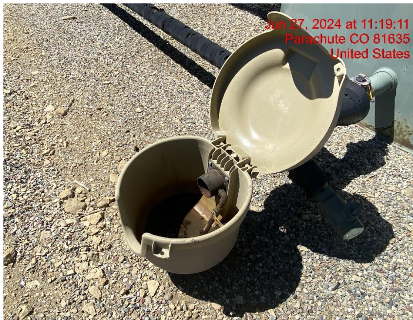
Open-Ended Load Line – Photo #01975
