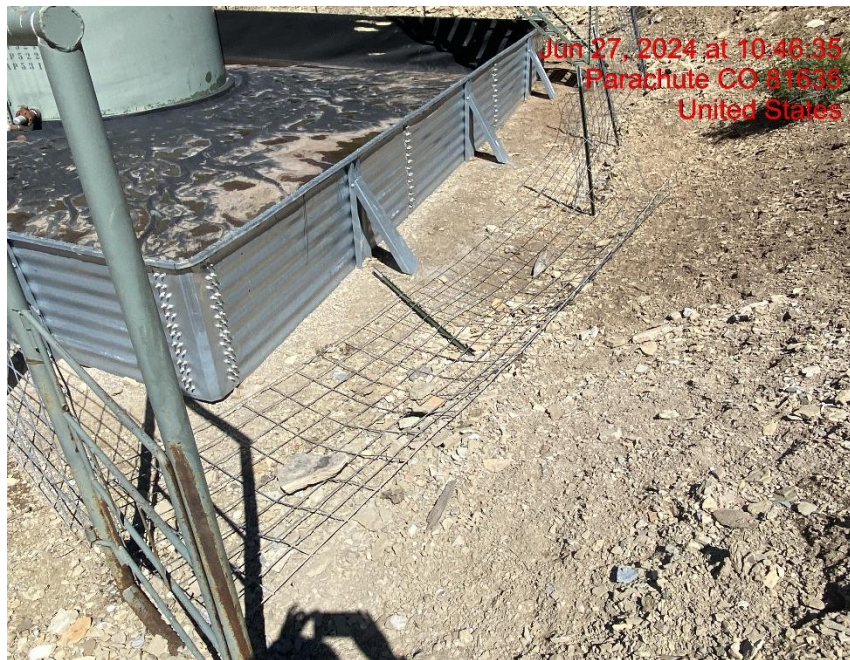
Insufficient Erosion Control/Site Degradation – Photo #01926
