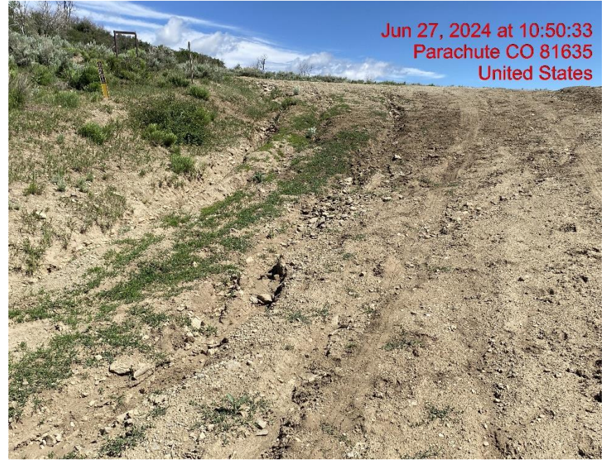
Insufficient Erosion Control/Rill Erosion Bypassing Ditch BMP on Access Road – Photo #01931
