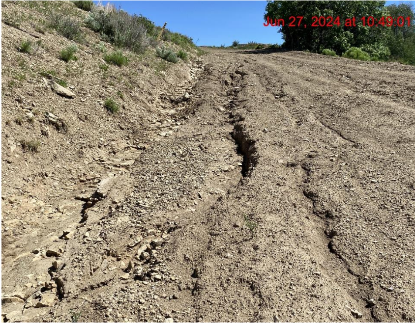
Insufficient Erosion Control/Rill Erosion Bypassing Ditch BMP on Access Road – Photo #01929
