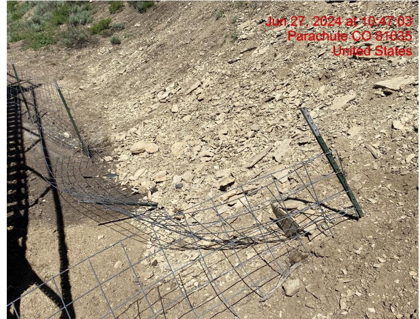
Insufficient Erosion Control/Site Degradation – Photo #01928
