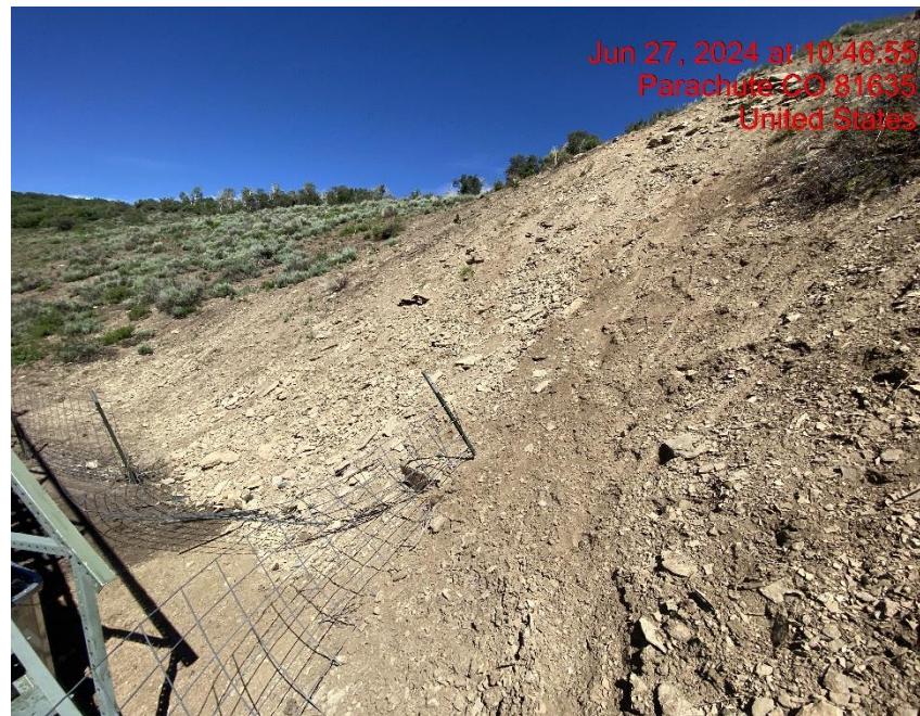
Insufficient Erosion Control/Site Degradation – Photo #01927
